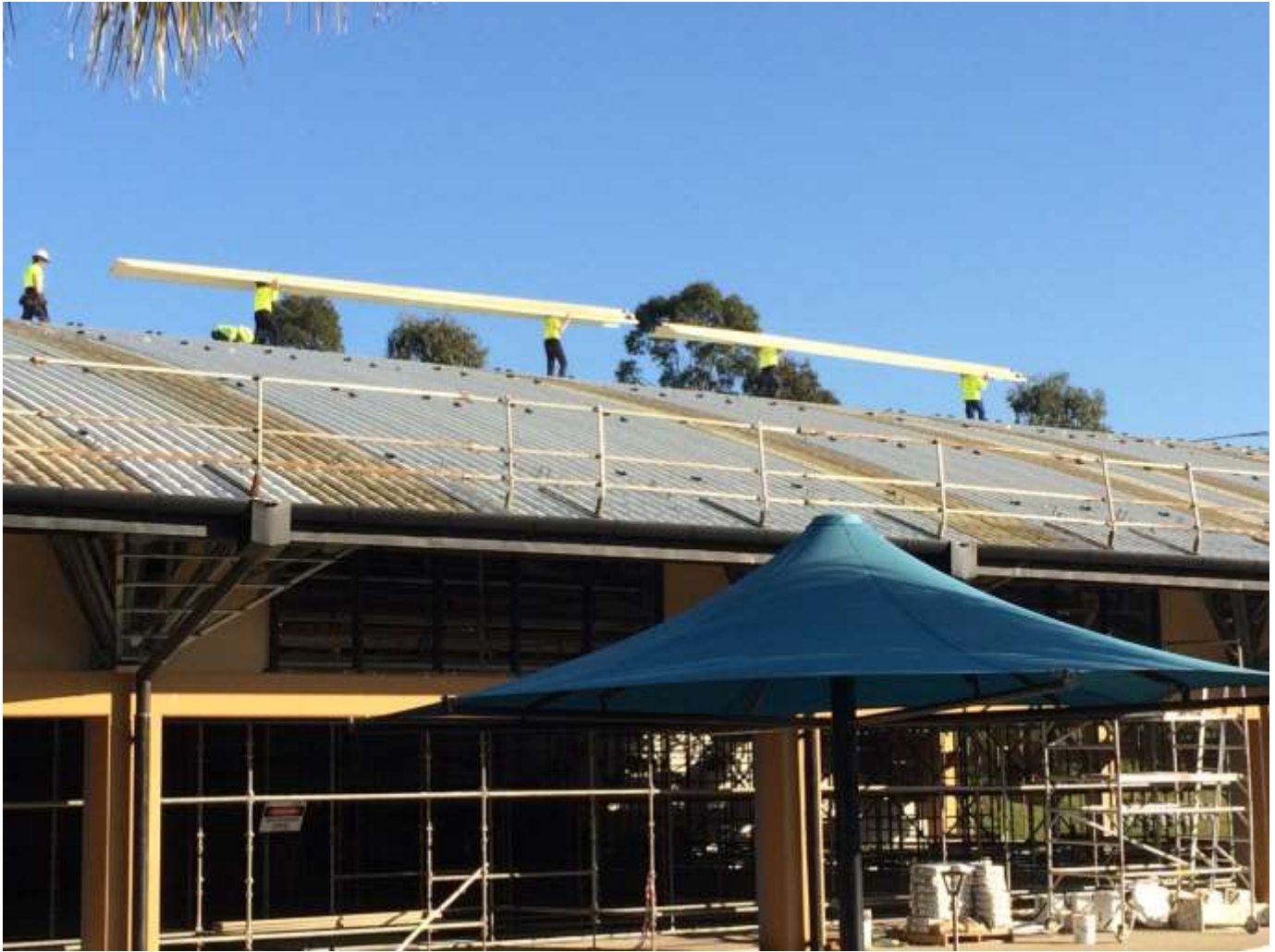
Clear sheeting to roof being removed
