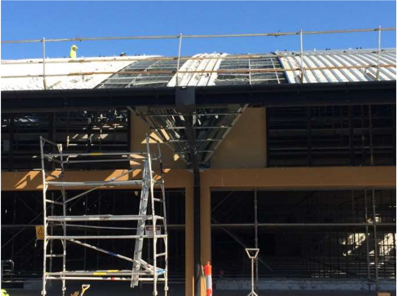
A section of the roof with the clear sheeting removed.
