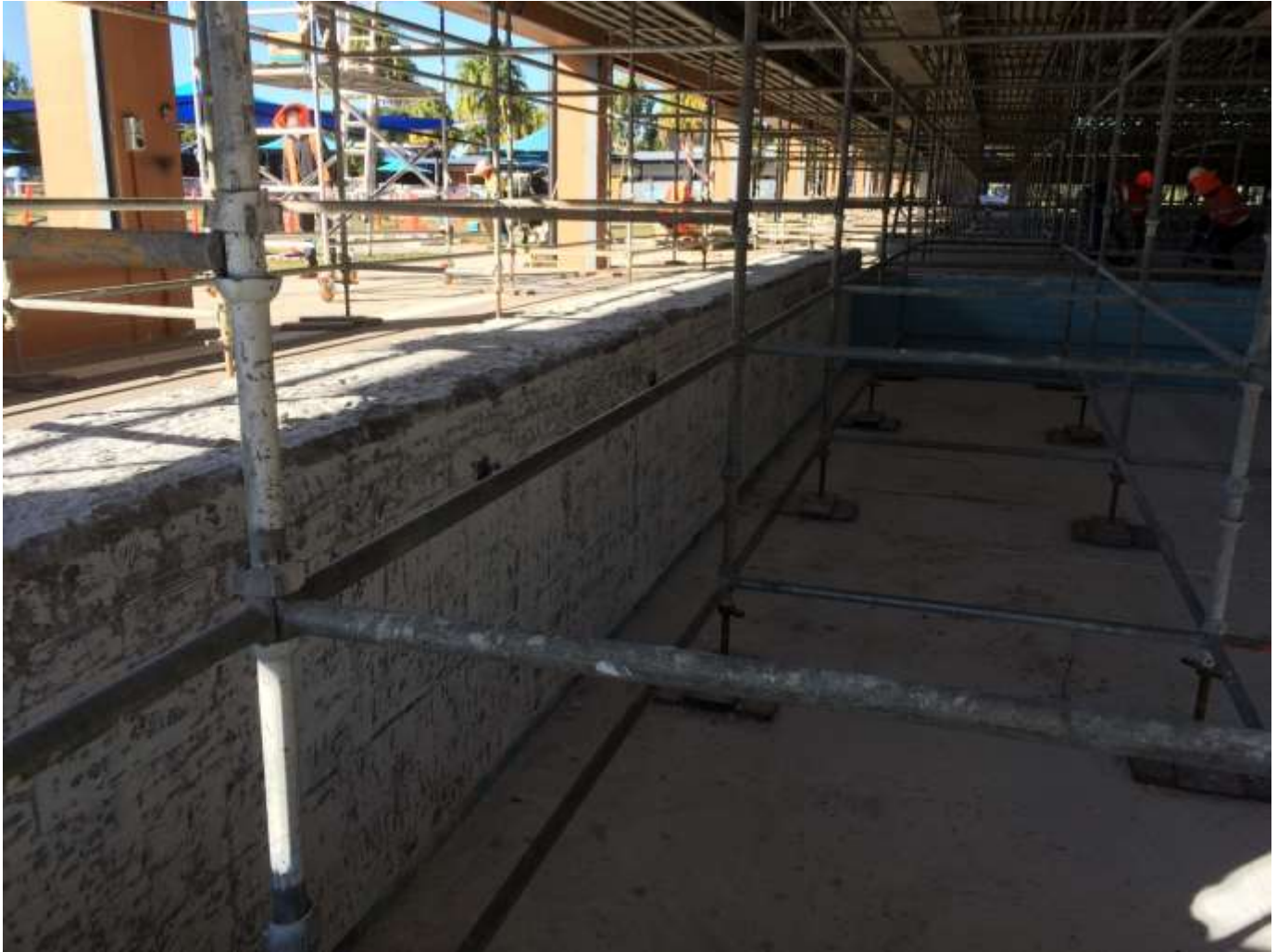
25m Pool (east side) - tiles removed to hob wall
