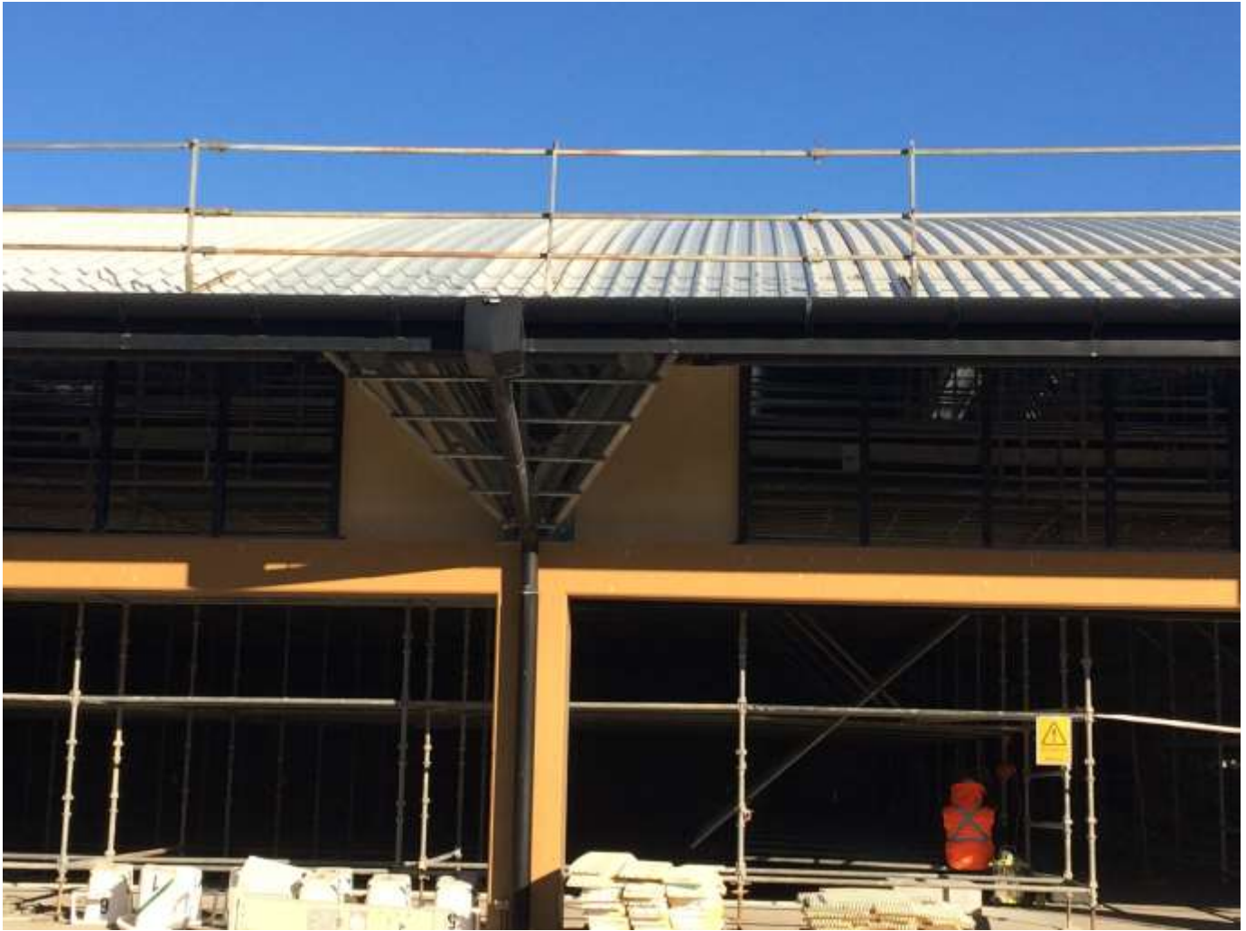
A section of the roof with the new clear sheeting installed
