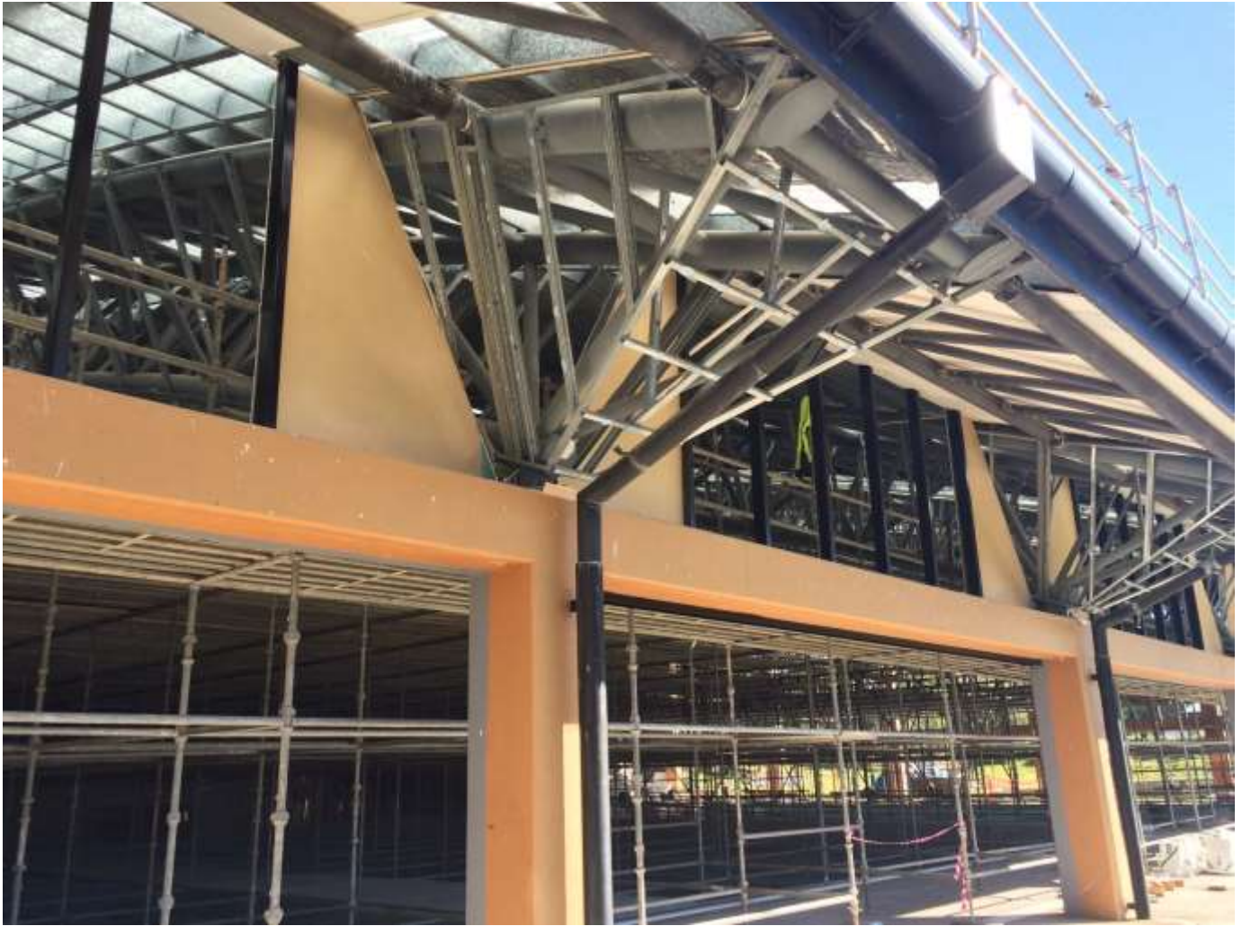
East face of building - new window frames being installed
