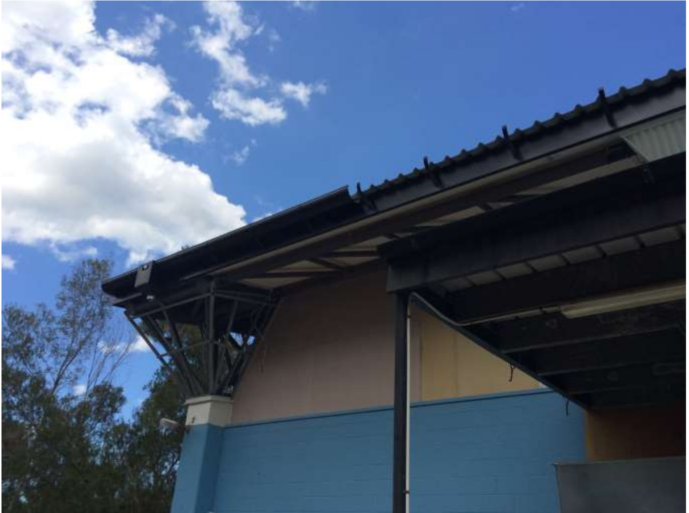
New gutter being installed to the rear west face
