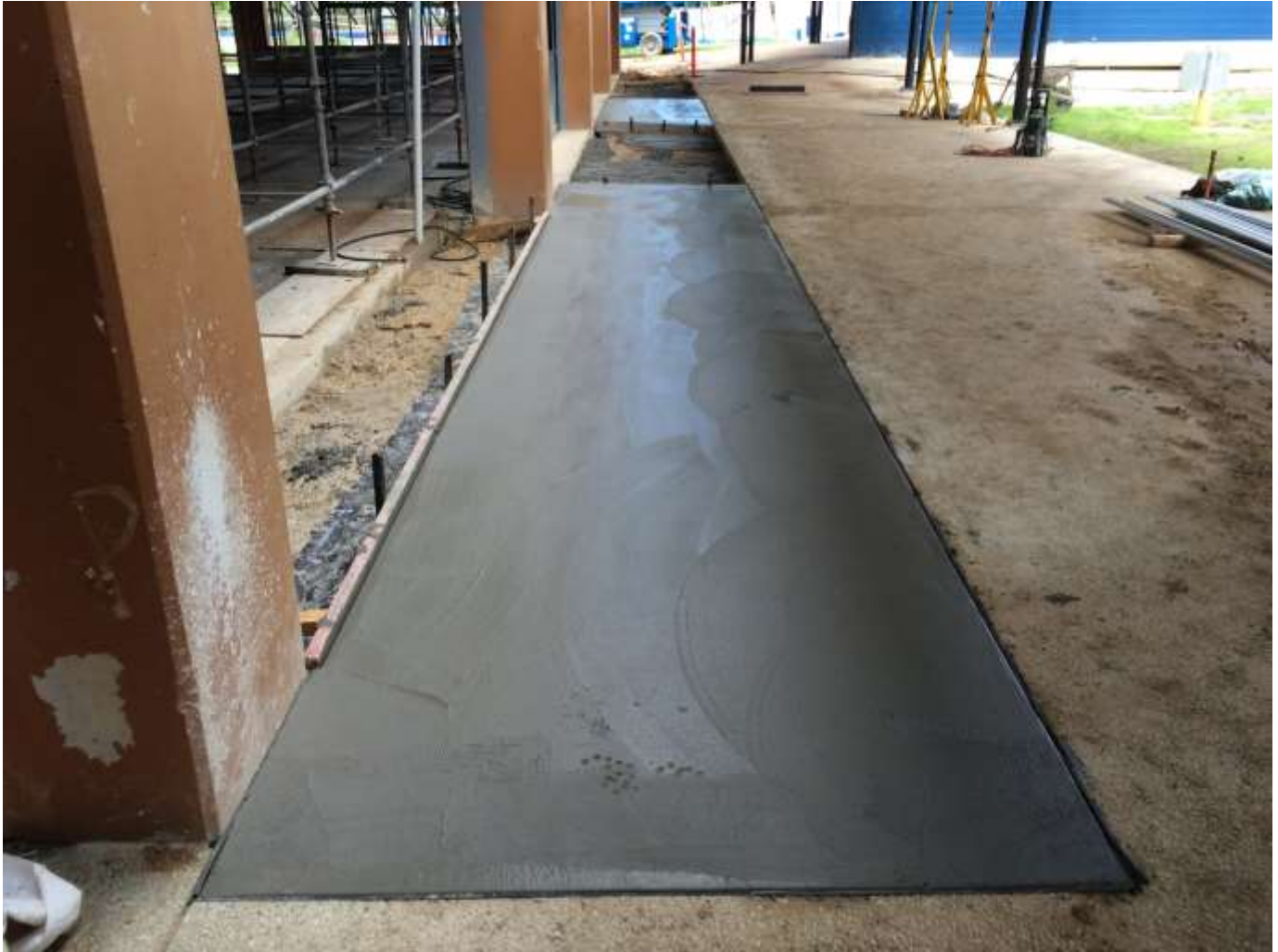
Paving being reinstated to the southern end of the building
