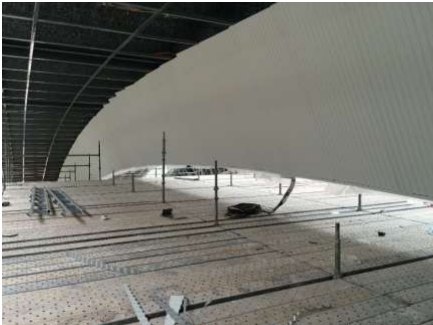
Ceiling truss lining being installed
