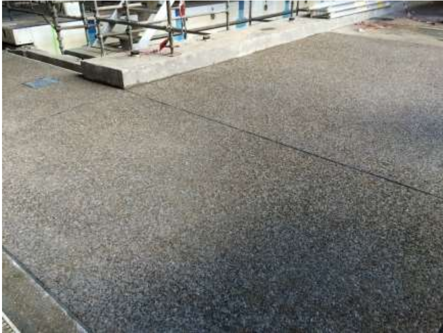
50m pool concourse reinstatement
