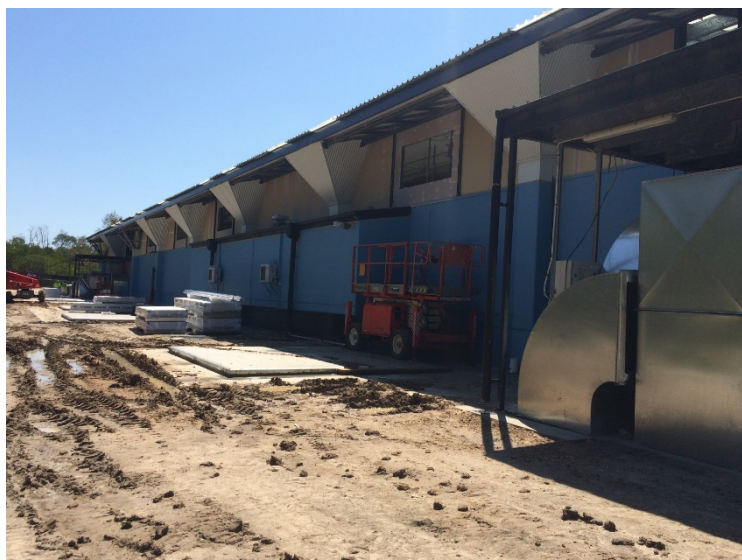
West (rear) wall - lining to truss end box outs and painting
