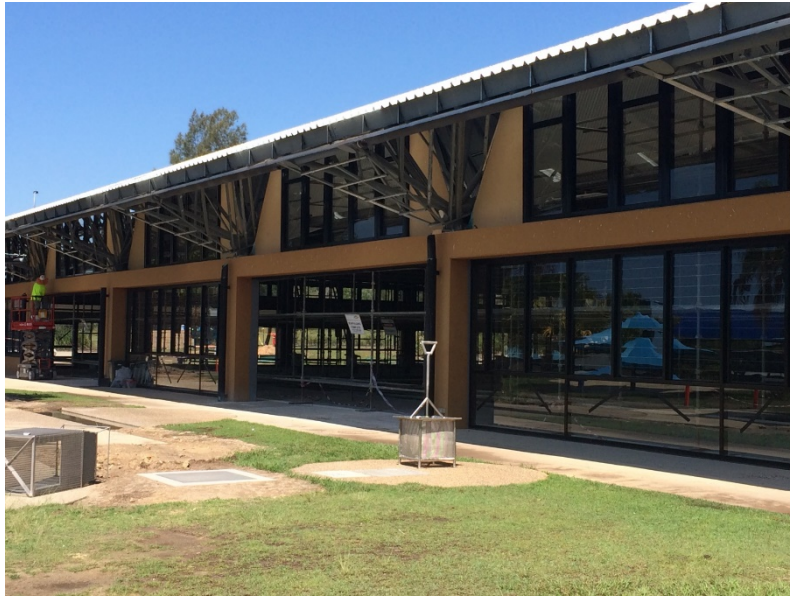
East wall - new fixed and louvre windows progressively being installed
