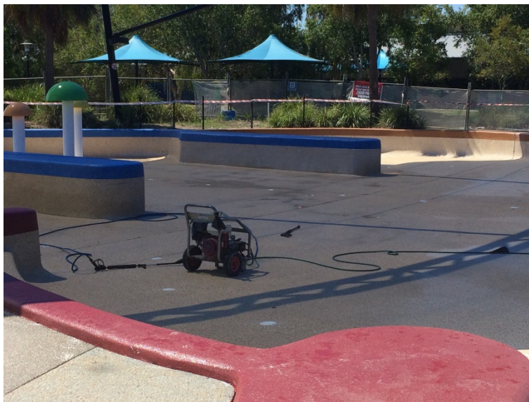
Leisure Pool - pool hob repairs complete
