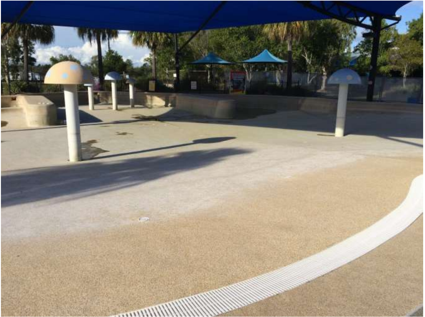
Leisure Pool - empty of water
