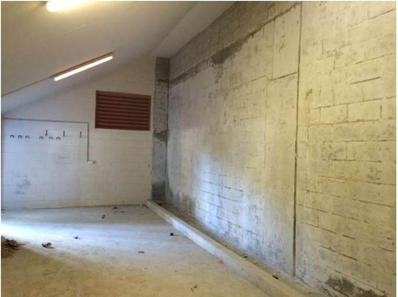
Store-room under grandstand - preparation for waterproof coating
