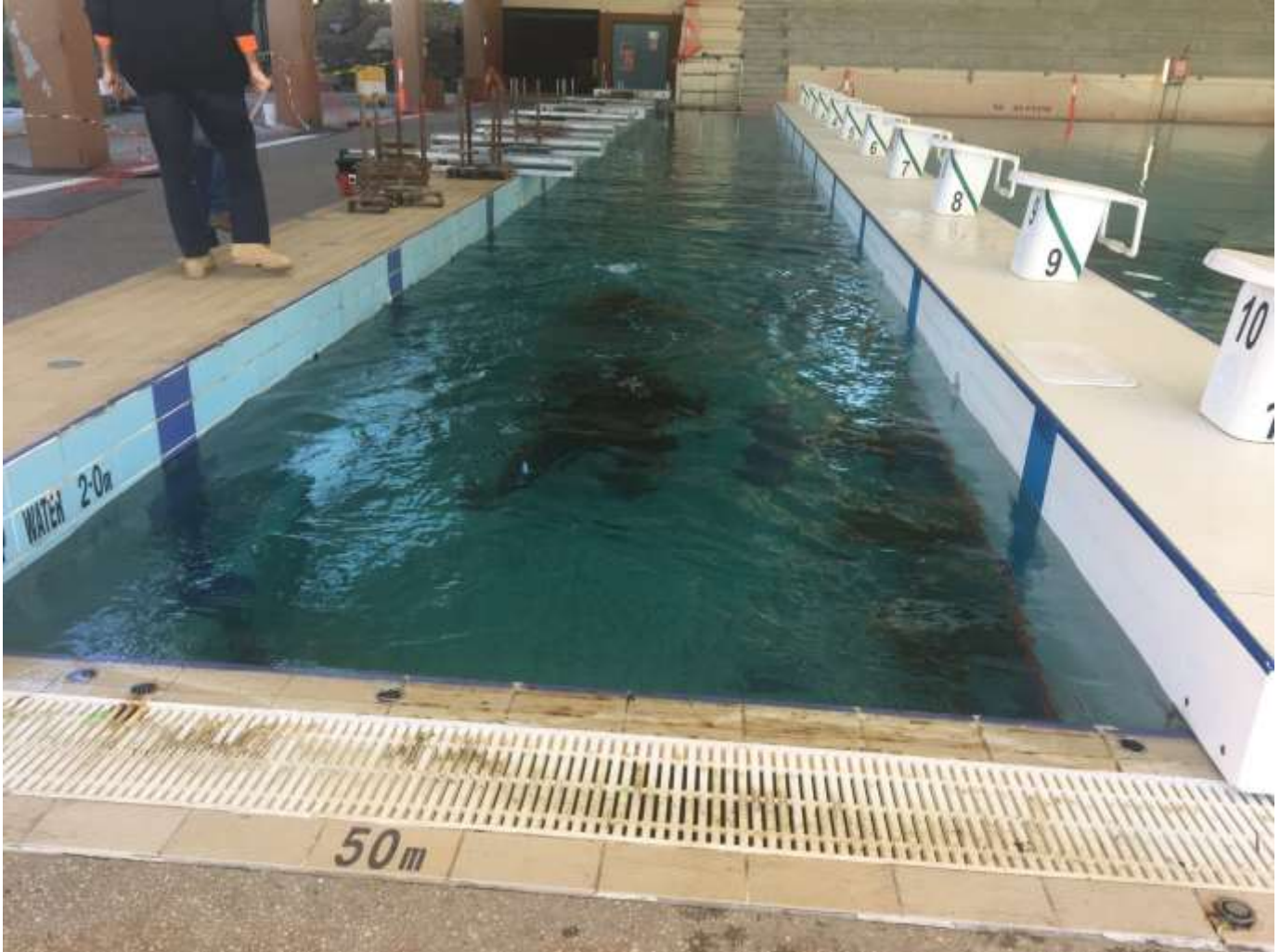
50m Pool - Divers installing scaffold support for the moveable bulkhead
