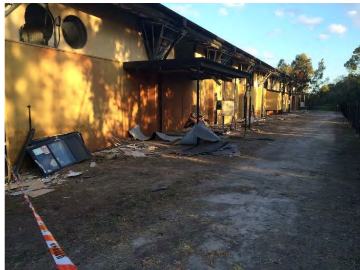
Image above: Ventilation plant removed to rear of building.
