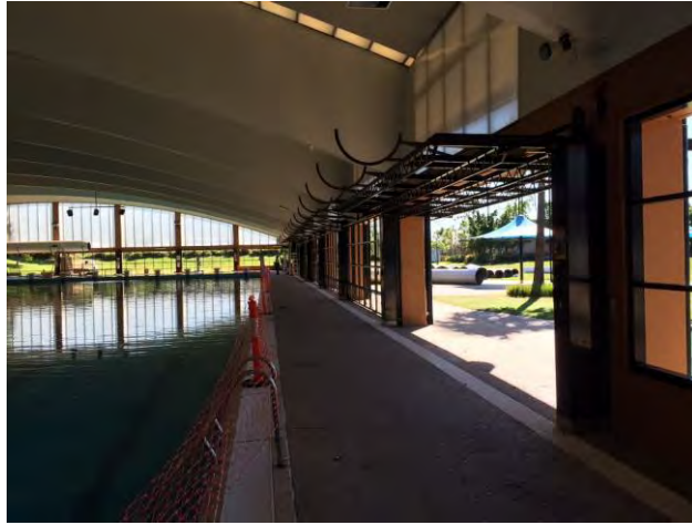
Image above: Demolition and removal of old ventilation systems.
