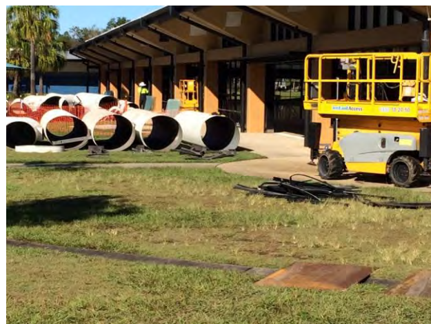
Image above: Ventilation system work removed from building.
