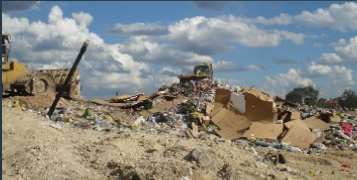
Landfill – making a new cell to fill
