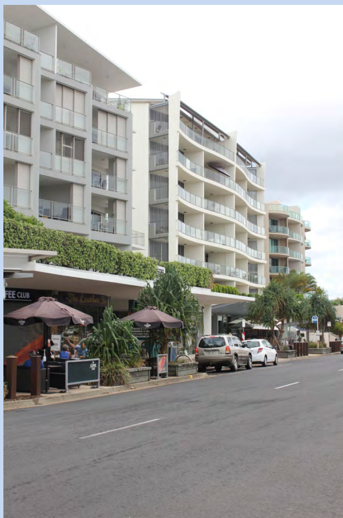
(Cotton Tree) Breaking a line of cars with kerb build-outs for landscaping, street furniture, outdoor dining or street trees.
