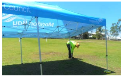
Walk marquee inwards until frame is 75% of full extension
