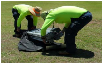
Fit the protective cover to frame. Fold roof & wall and store in Protective cover provided
