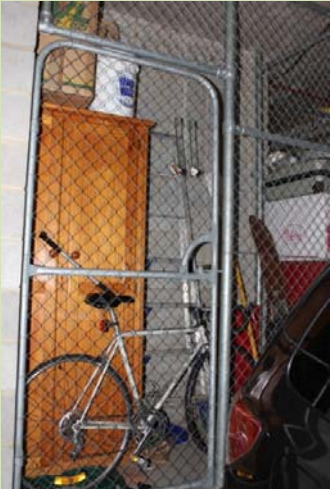
(Maroochydore) Storage space does not include bicycle parking and should be provided in addition to the required bicycle parking space.
