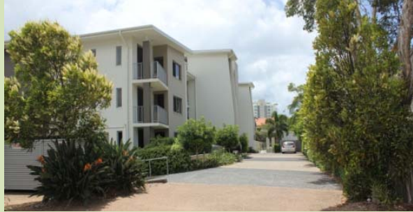
(Cotton Tree – side view. Vehicle access is from the secondary street frontage).
