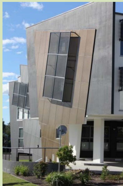
(Maroochydore) Building bulk and blank walls should be reduced through the use of architectural features, recesses and projections, balconies and variations in materials and finishes.
