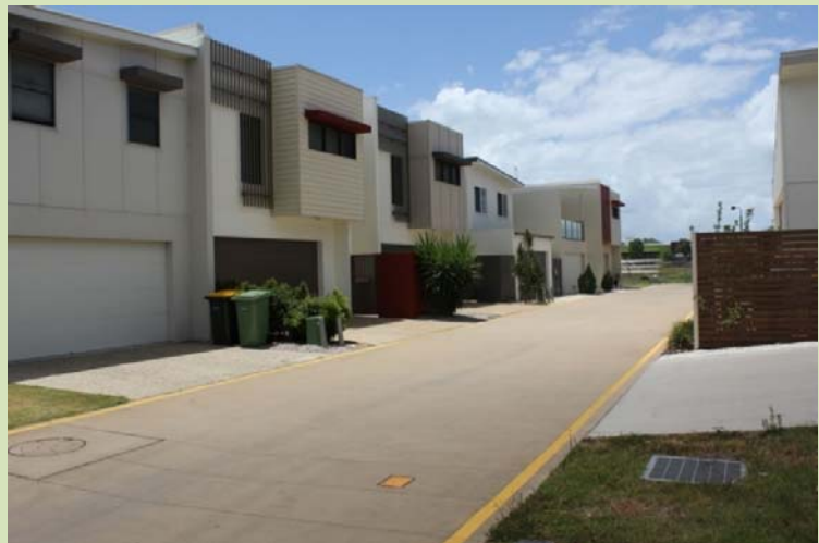
(Maroochydore) Rear – adjoining lane Lanes should reduce areas for concealment.
