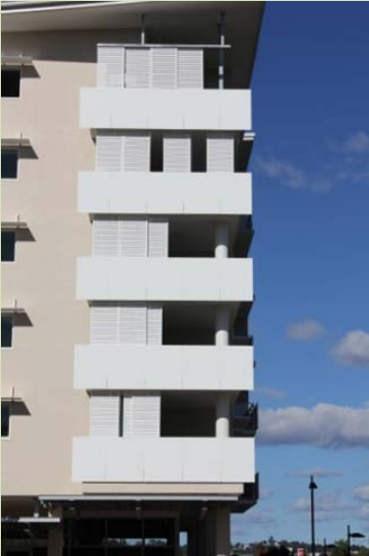
(Maroochydore) Provide balconies with operable screens, Juliet balconies or operable walls/sliding doors with a balustrade in specific locations where noise or high winds prohibit other solutions e.g. along rail corridors, on busy roads or in tower buildings.
