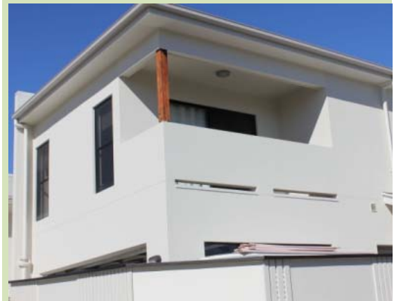
(Maroochydore) Solid balustrading can provide privacy to balconies whilst also facilitating surveillance.
