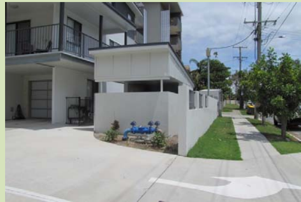
(Redcliffe) Covered bin storage areas should be well ventilated.
