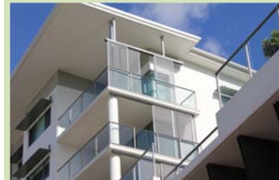
(Maroochydore) design solutions such as louvered screens with specific views, operable or fixed vertical louvres or planter boxes along the edge of balconies should be utilised to limit sight lines. Obscure glazing is the least desirable screening method for apartments.
