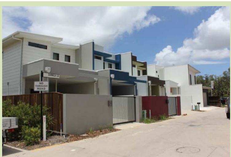
(Maroochydore) Rear – adjoining lane Fencing to a lane can be 1.8m high and 0% transparent to screen private open space and servicing areas.
