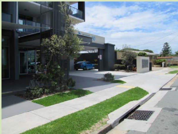
(Clontarf - Angled side view to see screening treatments) Mail collection, landscaping and an architectural feature forming part of the building all work together in this example to reduce the visual dominance of ground floor car parking areas.
