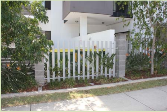
(Chermide) Bin storage areas are to be screened and aesthetically treated to not be overbearing or visually dominate the streetscape.
