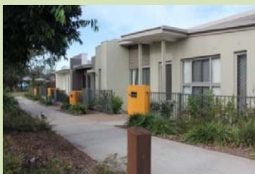
(Fitzgibbon) Front - adjoining park
