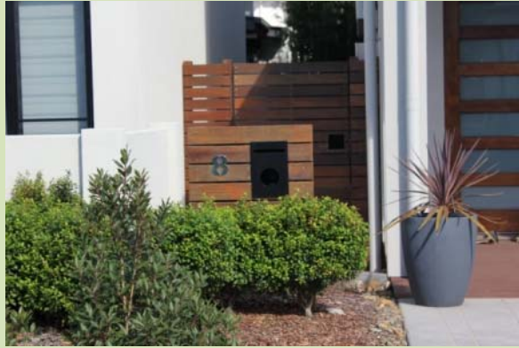
(Maroochydore) High fencing in line with the main building line with a gate can provide both screening for bin storage areas and ensure convenient access to collection point.
