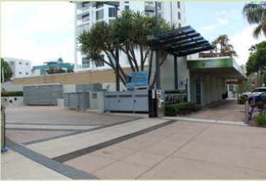
(Maroochydore) Utilities such as bin storage, booster pumps and electrical transformers should orientate along internal driveways, perpendicular to the street frontage.
