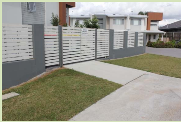
(North Lakes) Accessible to the collection point.
