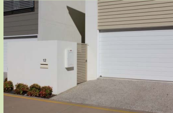
(Maroochydore) Visual clutter created by utilities should be screened in laneways.
