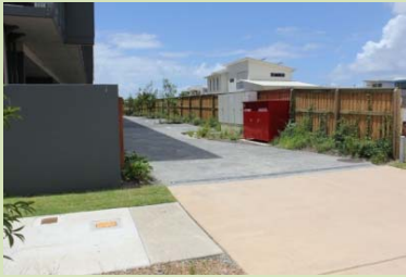
(Maroochydore) Services such as fire hydrants and electrical transformers should not be visually prominent at the streetscape. Screening and landscaping should be utilised to reduce the visual dominance utility areas have on the streetscape and adjoining sites.
