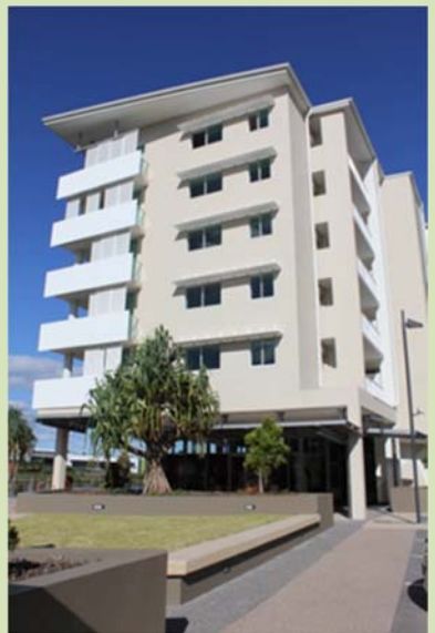
(Maroochydore) Mixed use buildings should open out onto public spaces e.g. streets, open space or plazas etc.
