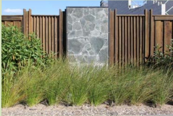
(Maroochydore) Where solid fences are unavoidable they should include variation in material, reduce flat surfaces and incorporate landscaping in front to reduce visual dominance and assist in the prevention of graffiti.
