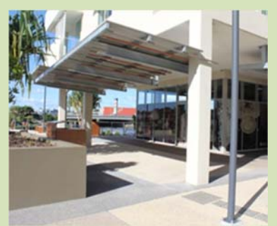
(Maroochydore) Awnings and street furniture can be added once the ground floor is converted to a non-residential use.
