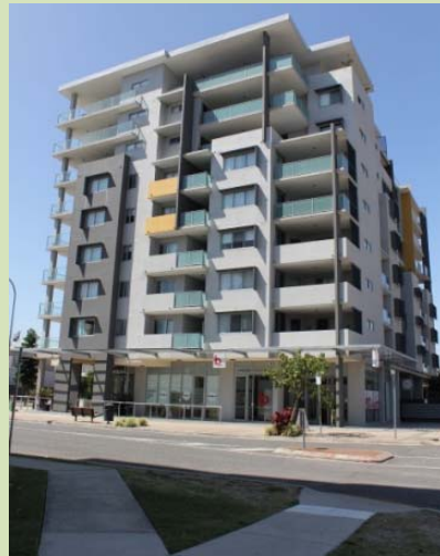
(Chermside) High buildings provide vertical articulation through a distinct top, middle and base section.
