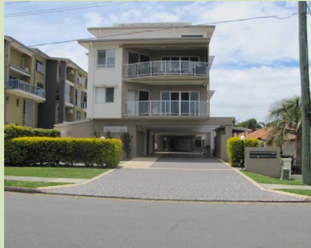
(Margate) The above example uses an architectural feature forming part of the building as a way of screening ground floor parking areas.
