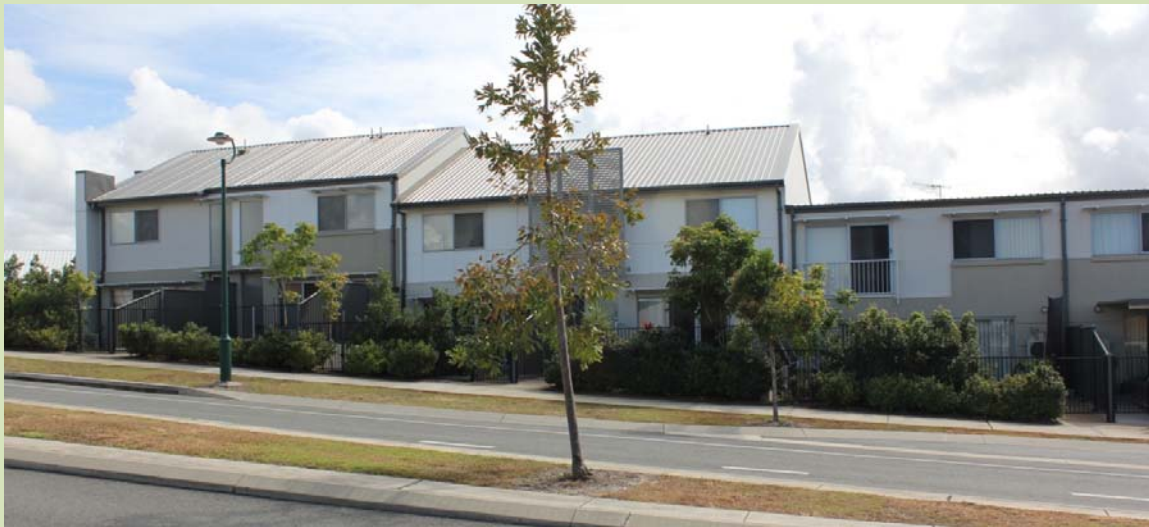
(North Lakes) Stepped terrace housing
