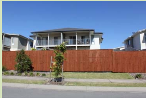
(Maroochydore) Solid front fencing that is higher than 1.2m dominates the streetscape. The example above would be improved by bringing the building forward, locating private open space to the side or rear and having a solid fence not exceeding 1.2m in height with a pedestrian gate.
