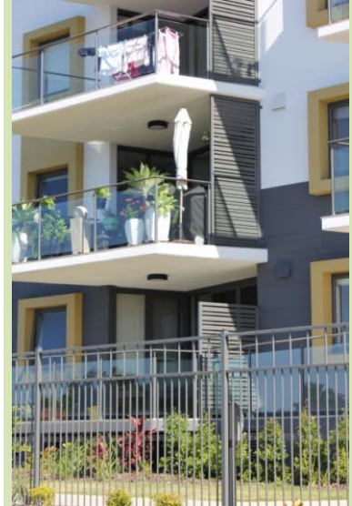
(Kawana) Where balconies are used to house equipment and plant such as clothes drying, air conditioners etc. this equipment should be screened.
