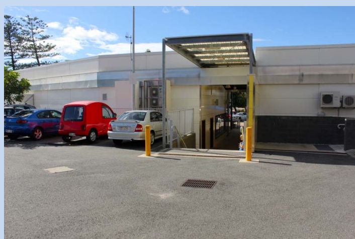
(Coolum) Access to main street from rear car park.
