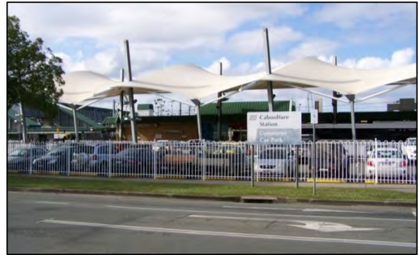
Entrance to Caboolture Station from Matthew Terrace
