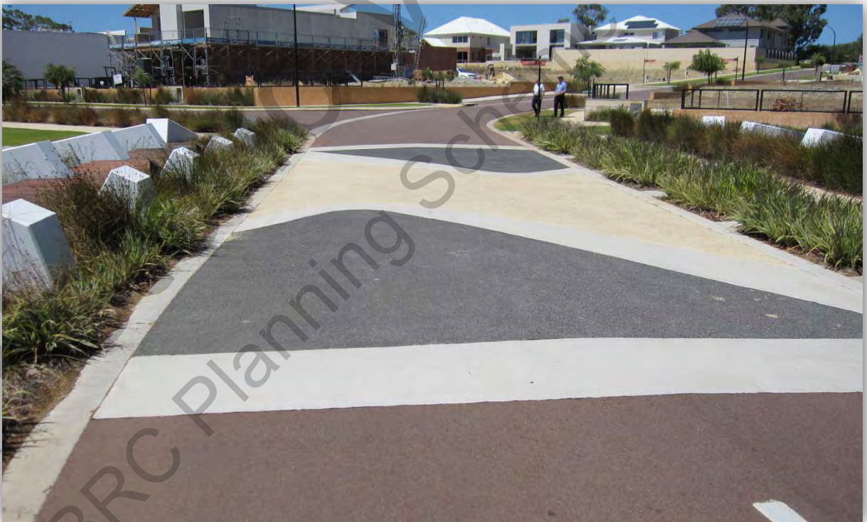
"Interference Patterns" create static spaces within the street and promote slower vehicle speeds
