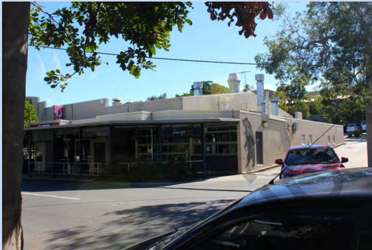
(Bulimba) Shared driveway providing access to shared car parking area at the rear
