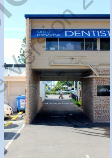
(Coolum) View from a lane through to a main street. Windows overlooking lane.
