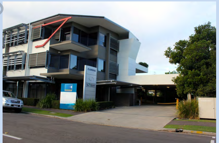
(Maroochydore) At grade and multi-storey parking located behind the building.
