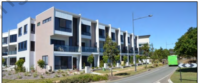
The 3 storey buildings above are town houses that can be easily converted to offices (North Lakes).
