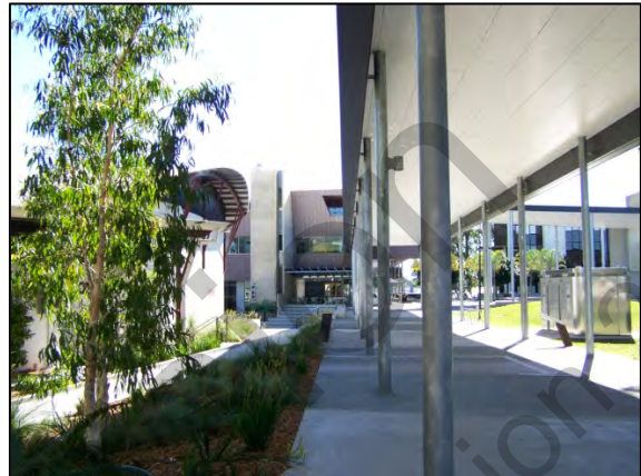
The Community Centre is on the left of this picture
