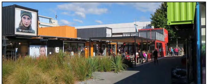
A temporary shopping arcade built from shipping containers (Christchurch).
