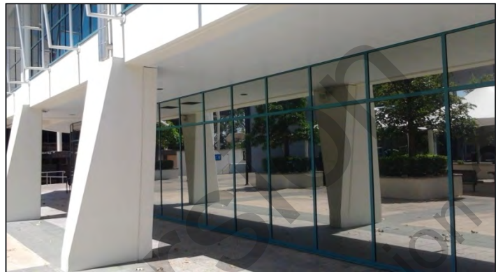
33 King Street, facing the town square
