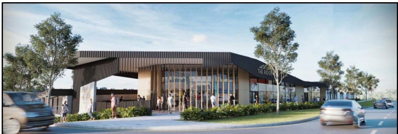
Figure 2: Streetscape perspective of Development Approval DA/2021/1179 from the corner of Morgan Road and Callaghan Road
