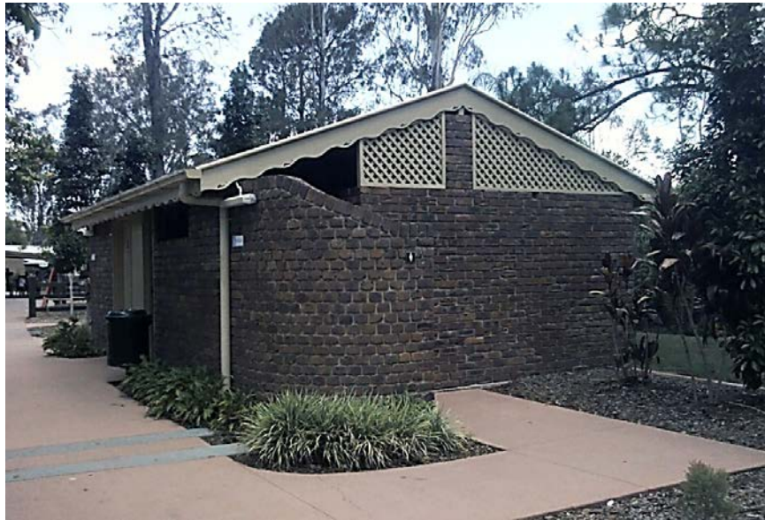
Figure 2 - Existing Amenities at John Scott Park
