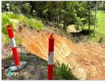
result of the 2022 floods. The eroded embankment will be reinstated and repairs to the roadway carried out to renew access and provide increased safety for road users.
