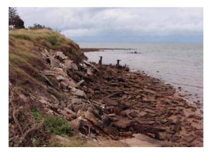
Figure 3-2 Uncoordinated armouring of the foreshore near "Gayundah" wreck
