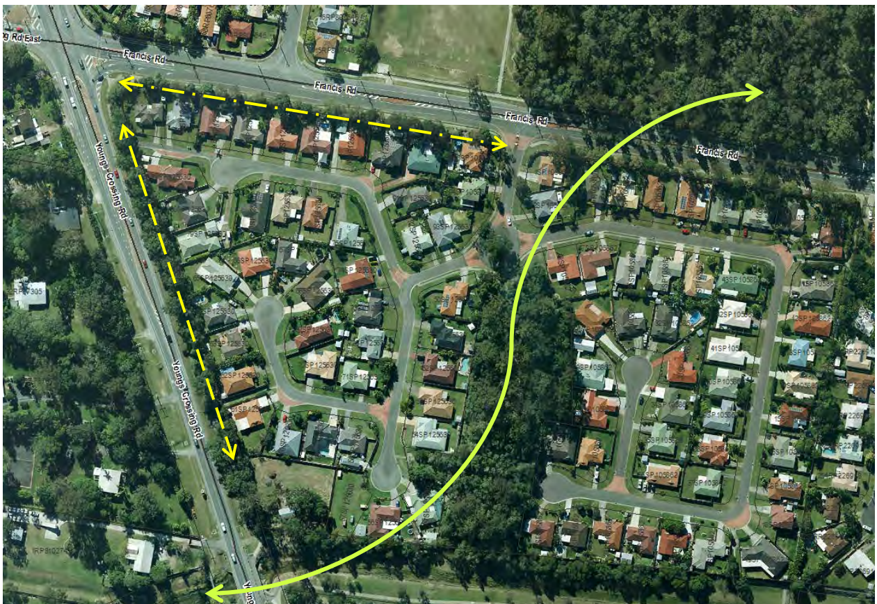
Tree retention along Young's Crossing & Francis Roads at Joyner; providing green linkages for animal movement (particularly koalas), shade for pedestrians and pleasant visual amenity.
