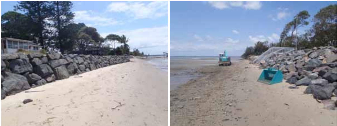
Figure 1-3 Rock Revetment Seawalls at Beachmere: Tightly Packed (left) and Loosely Placed (right)
