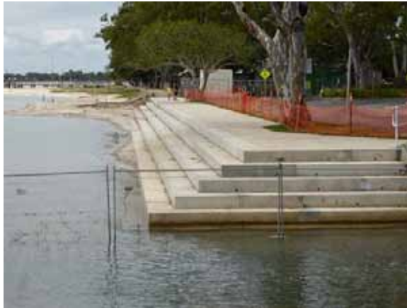
Figure 1-2 Precast Concrete Stepped Seawall at Bongaree (Auzcon, 2014)
