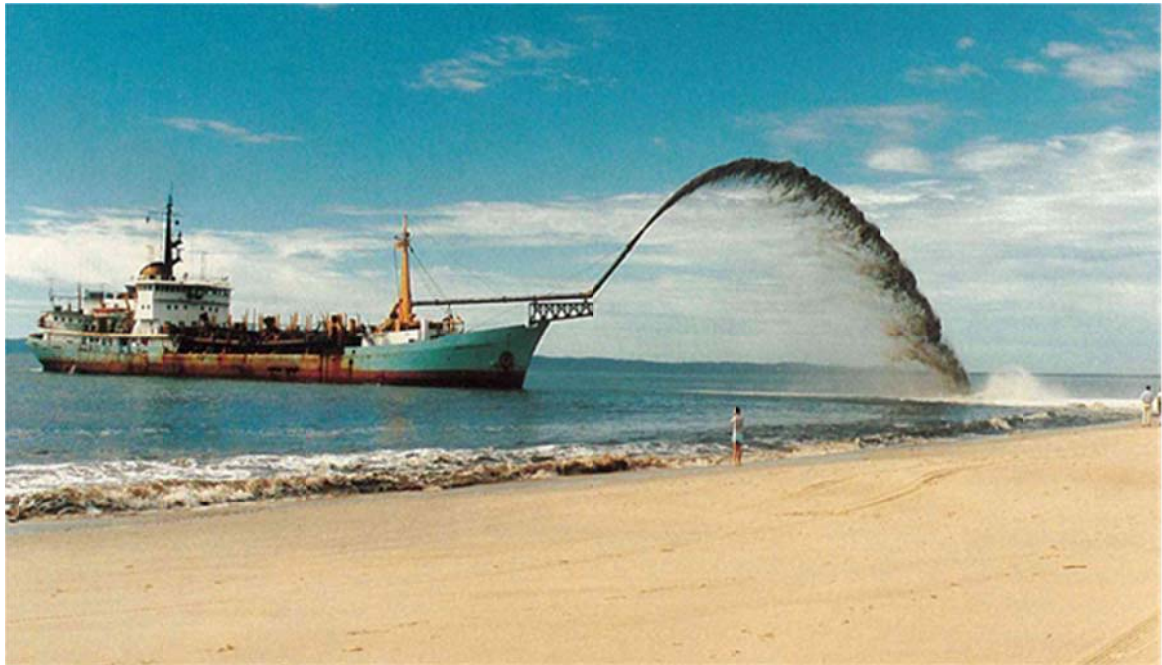
Figure 3-7 Nourishment Sand being Delivered ‘over-the-bow’ to Woorim Beach
