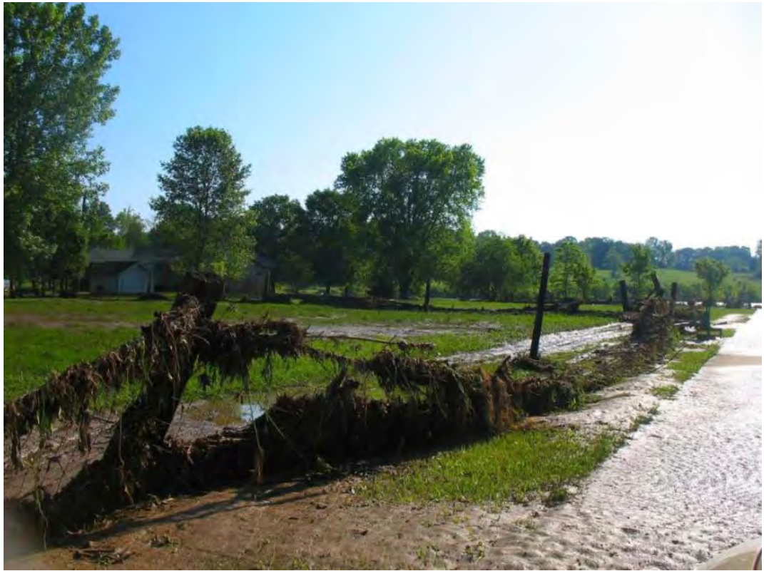
■ Figure 8-2 Fence Blockage Example
