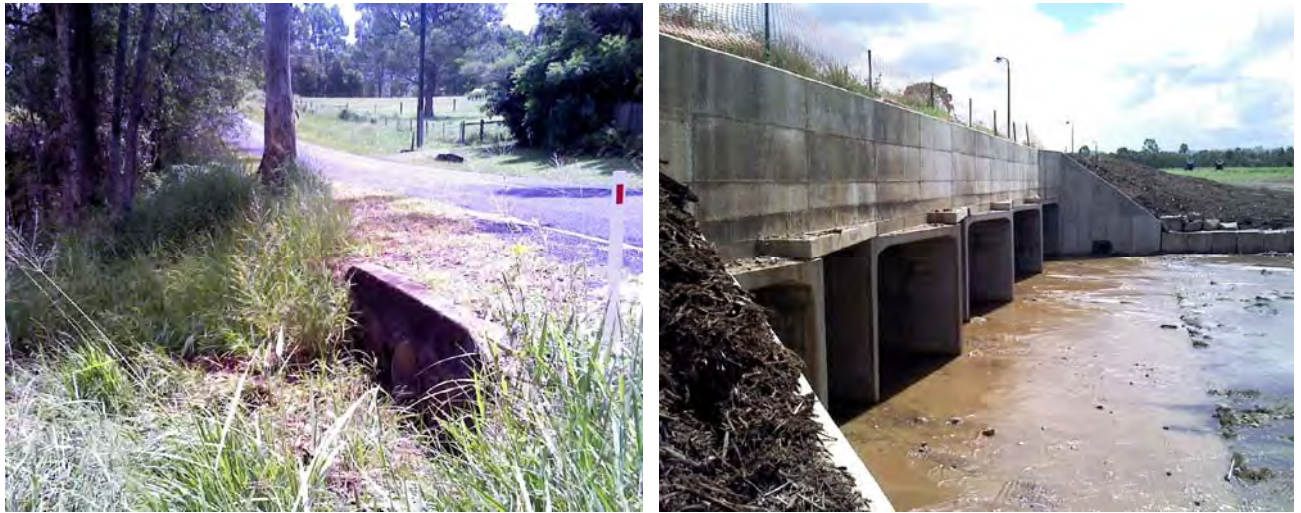
Image 3- 1 Photos of Small and Large Culverts with Blockage Applied
