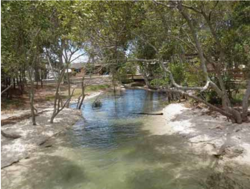
Photo Plate 7-1 Culverts under road beside boardwalk
