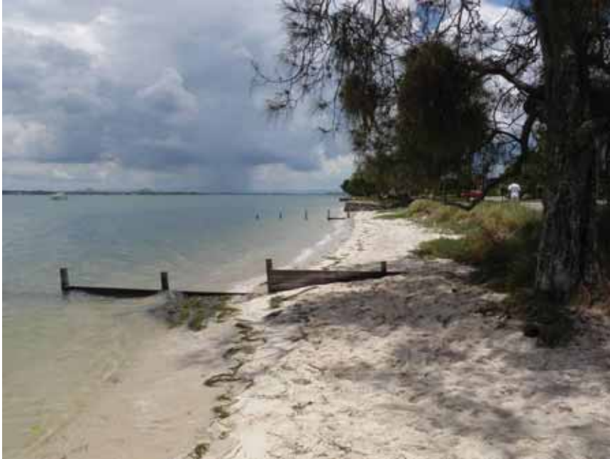
Photo Plate 7-3 Northern Sylvan Beach with timber groynes
