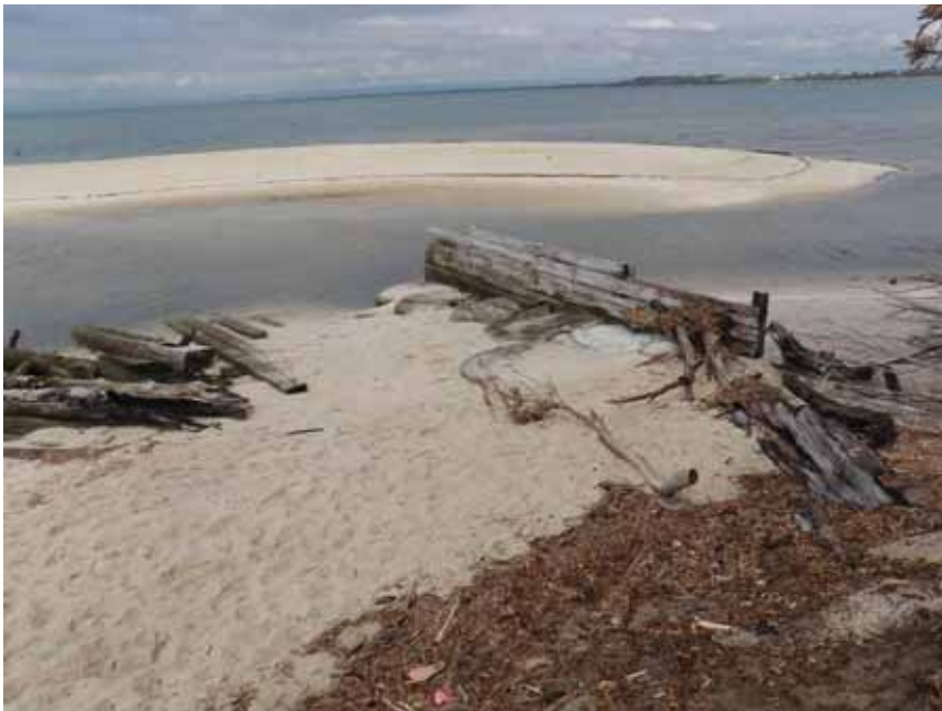
Photo Plate 3-4 Timber groyne and other structures at mouth of channel
