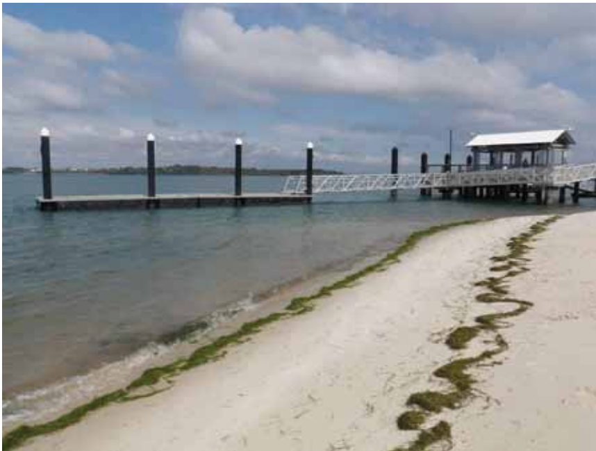
Photo Plate 3-10 Sand build-up south of Bongaree Jetty
