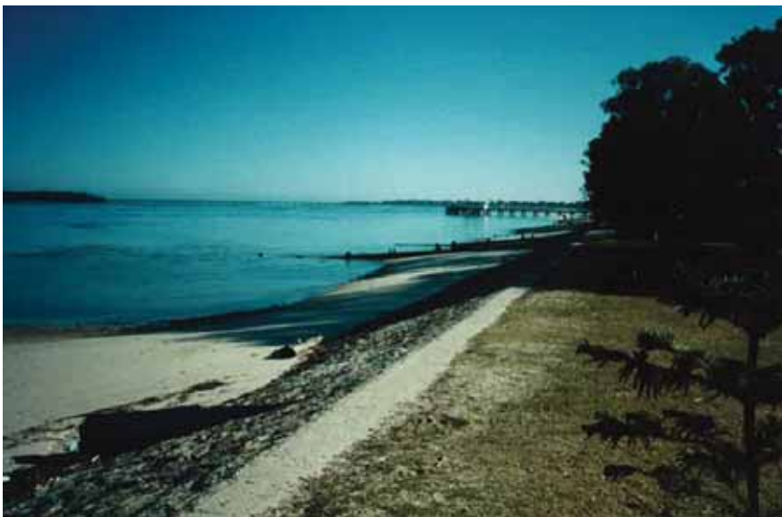
Photo Plate 3-8 Seawall north from timber groyne 1990s
