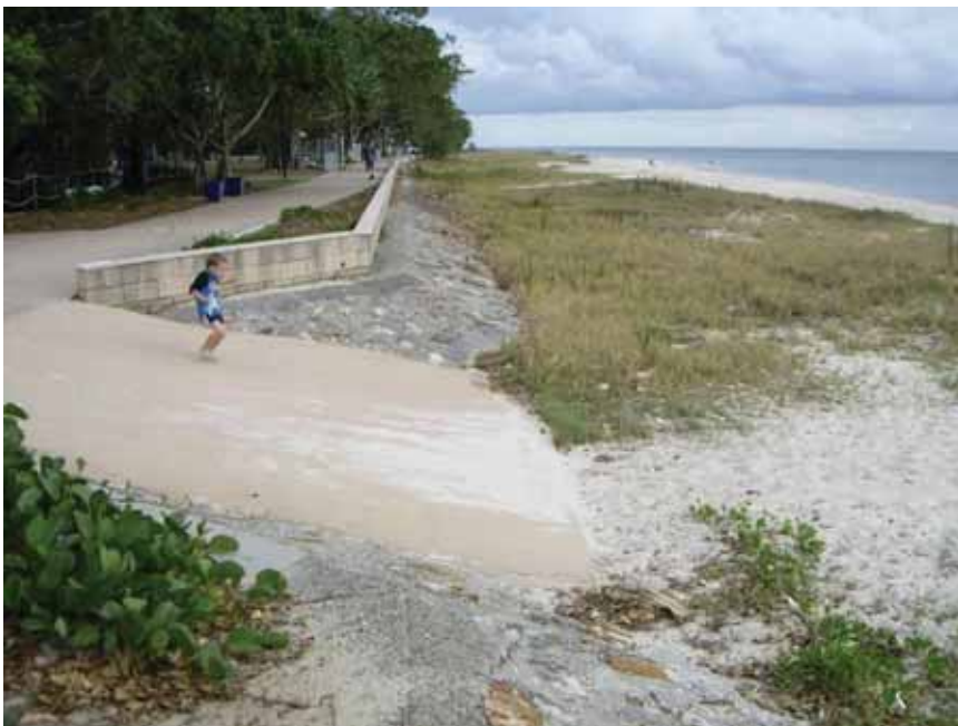
Photo Plate 3-6 Seawall and foredune south of Bongaree Jetty
