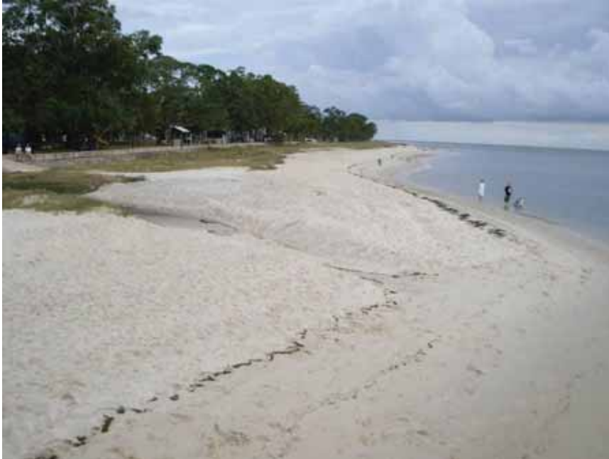
Photo Plate 3-9 Stormwater outlet south of Bongaree Jetty
