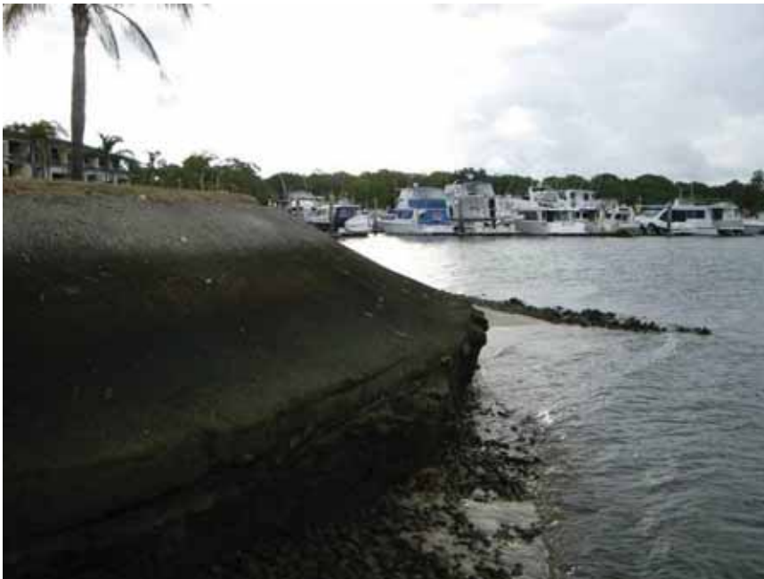
Photo Plate 9-4 Sea wall on southern side of marina entrance
