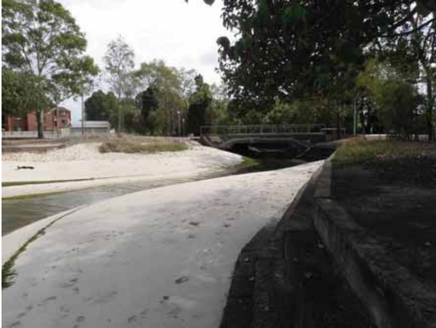
Photo Plate 4-3 Shirley Creek bridge and seawall structures
