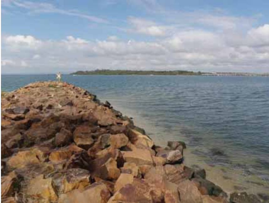
Photo Plate 4-7 Bribie Gardens Estate groyne structure in the canal
