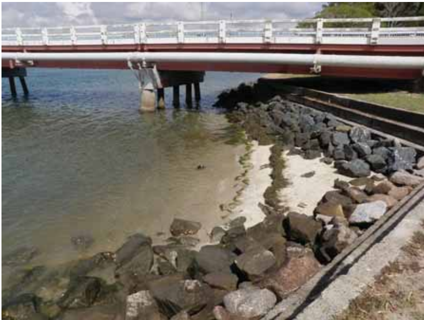
Photo Plate 5-4 Bribie Island Bridge
