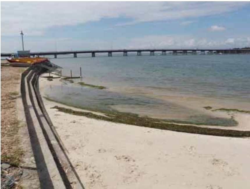
Photo Plate 5-6 Infrastructure north of bridge
