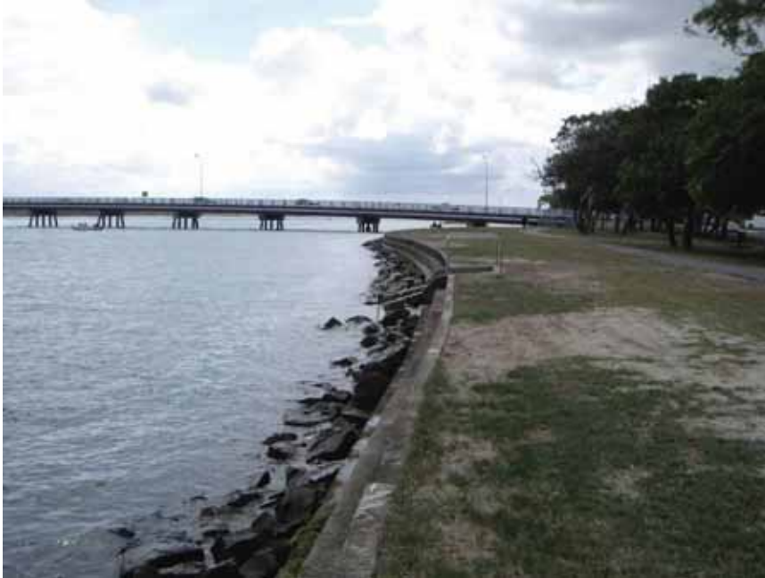
Photo Plate 5-3 Sea wall and rock protection south of bridge
