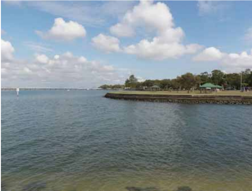
Photo Plate 5-1 Bribie Gardens Estate canal northern entrance
