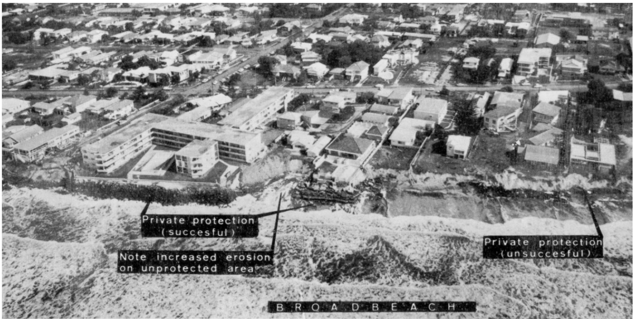
Figure 9.2 End Effects of Seawall (top) and example of successful and unsuccessful seawall terminations for private residences on the Gold Coast (bottom) (reproduced from WRL, 2012)
