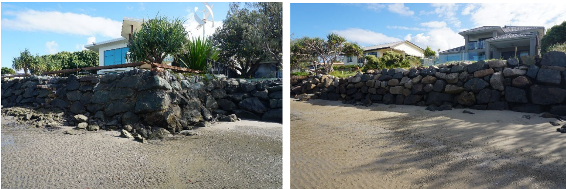
Figure 4.1 Examples of near-vertical gravity type seawalls comprised of placed boulders with mortar (left) and without mortar (right)
