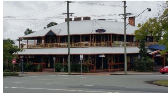
Woodford Village Hotel is located on a prominent corner and successfully contributes to the visual interest and traditional rural township character of Woodford.
