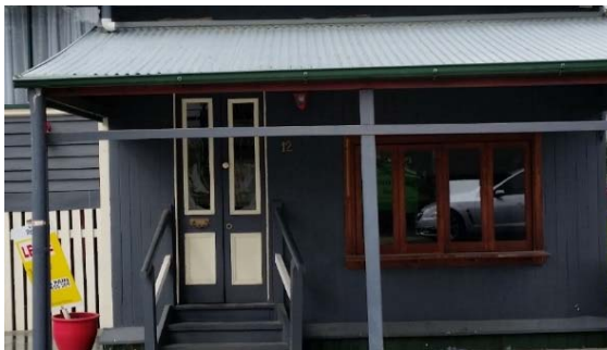
Examples of preferred window and door detail styles. Doors are normally inset with a small landing, as shown in both examples above.
