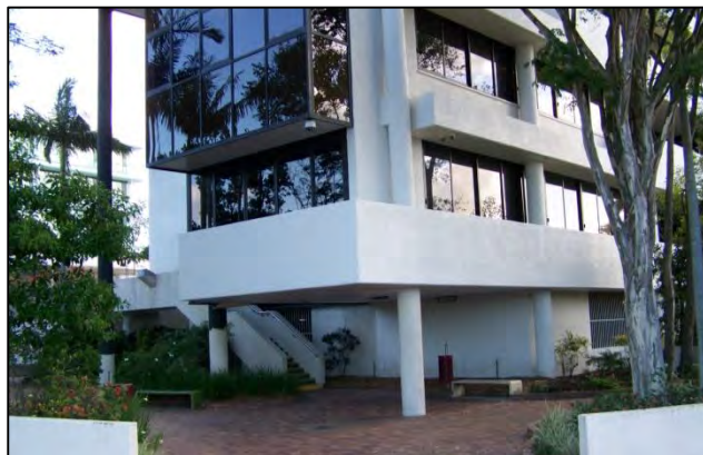
Façade facing onto plaza and Beerburrum Road
