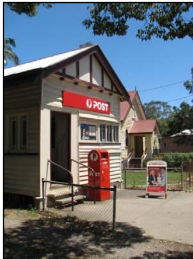
An example of wall/façade signage located above the building entrance.
