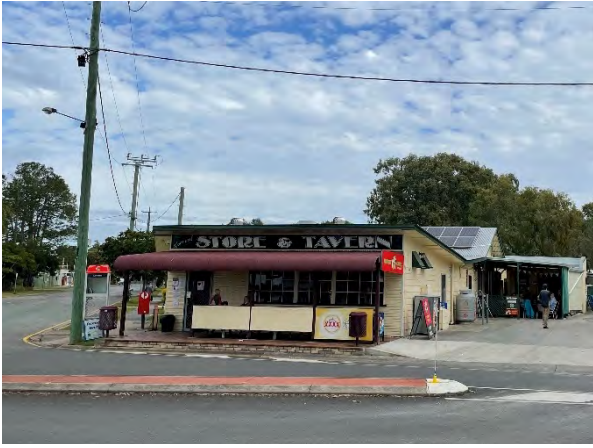
Toorbul store illustrates traditional colours and materials with its timber weatherboards and corrugated iron awning
