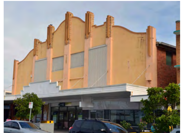
Decorative parapets in an Art-Deco style
