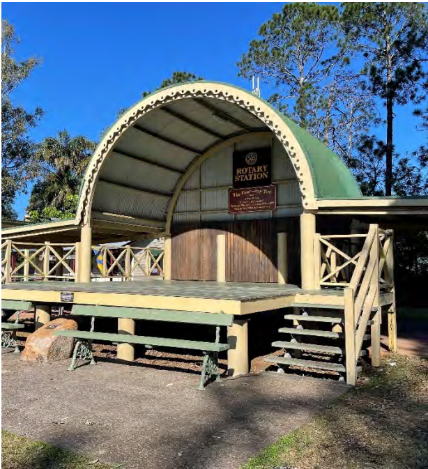
John Scott Park is the heart of the Samford Valley township and includes the 'Rotary Station' stage built with traditional materials and details.
