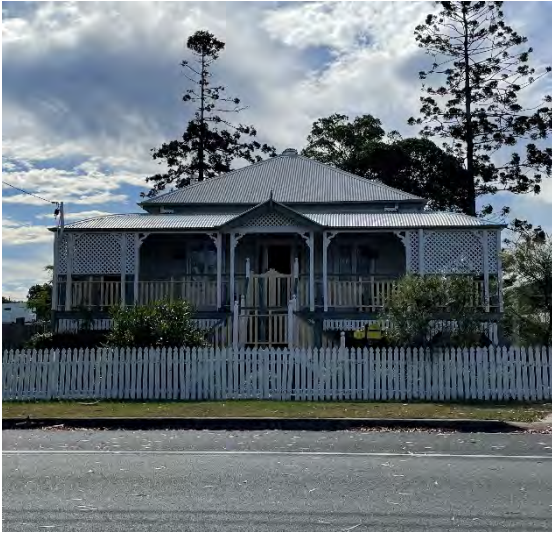
Traditional character homes with detailing, verandahs and screening.
