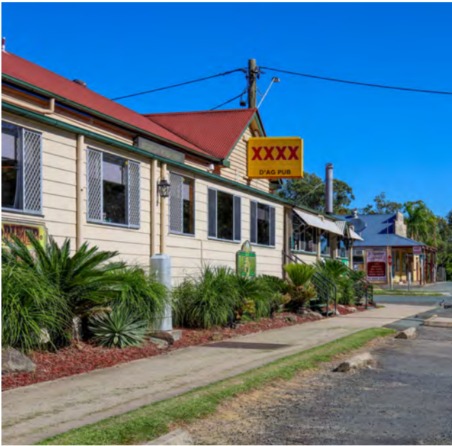
The 'Dag Pub and Motel' exhibits traditional colours and materials with its timber weatherboards and corrugated iron roof
