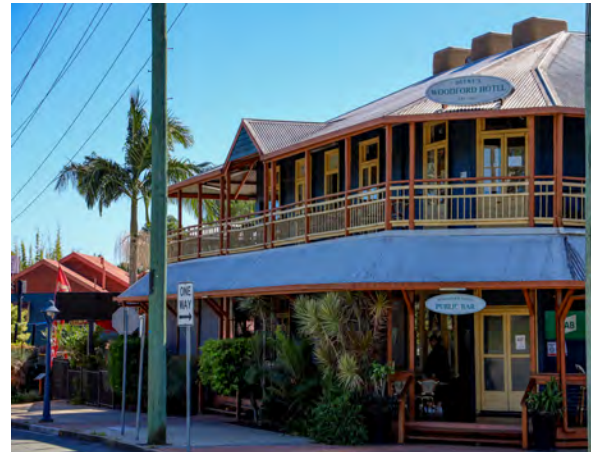
Character 'Queenslander' buildings with traditional colours, materials and moderately pitched roofs with narrow, decorative gables.
