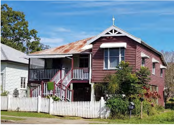
'Timber-and-tin' dwellings with traditional built forms, materials, colours and details.
