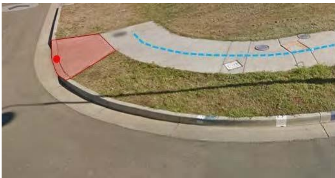
Figure 5: Pathway (blue) spatial representation with reference to a pram ramp (red polygon) and its spatial representation (red point) in the case where the pathway ends at the pram ramp.
