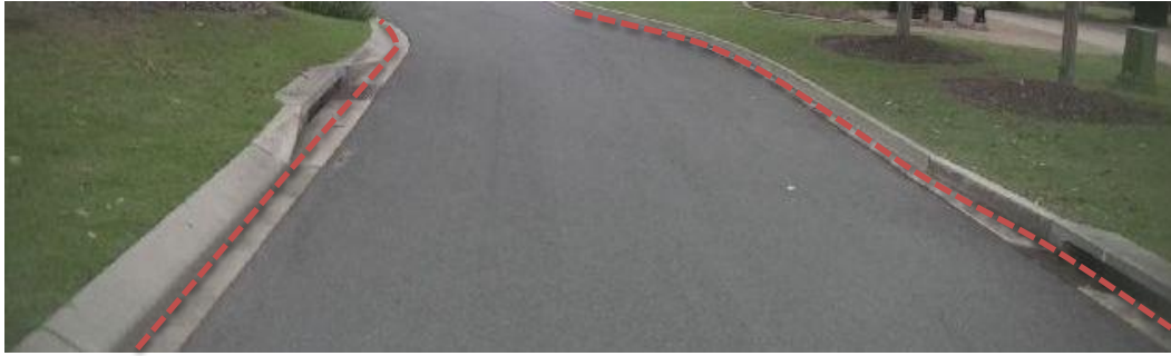
Figure 9: Kerb should be captured at the nominal kerb line as defined by IPWEA Standard Drawing RS-080. The above shows an example of where this would be for different kerb types.
