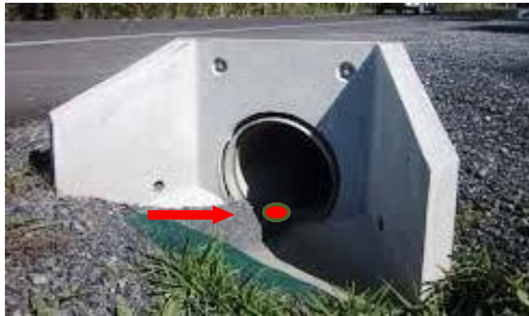
Figure 12: End structure point represents the invert of the headwall or end wall.
