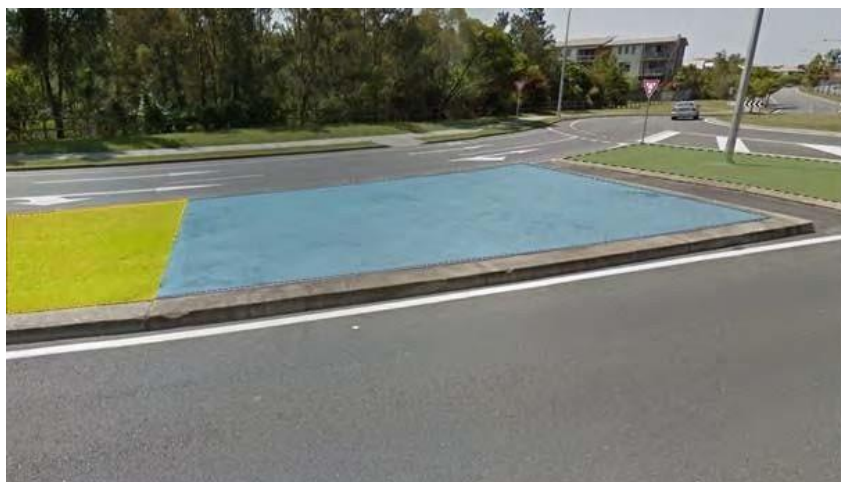
Figure 10: Road island capture is based on physical characteristics. Separate polygons are required when the type of island or infill material changes, as shown by the yellow, blue and green polygons above.
