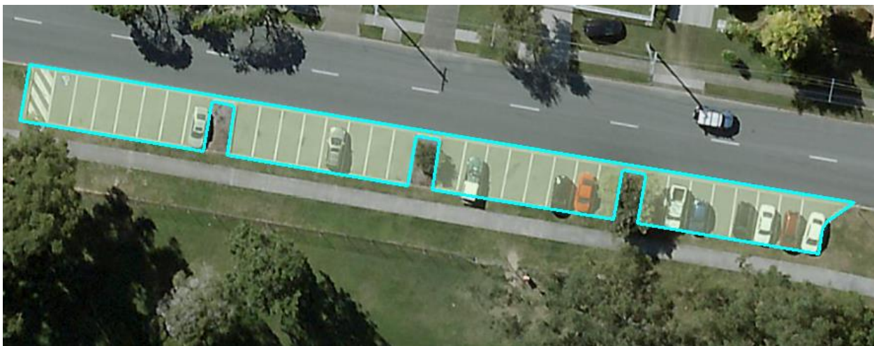
Figure 4: On Street Parking is separated from the road pavement by a change in materials or a physical barrier such as an invert kerb. The parking here is outlined in blue and contains one disabled space.
