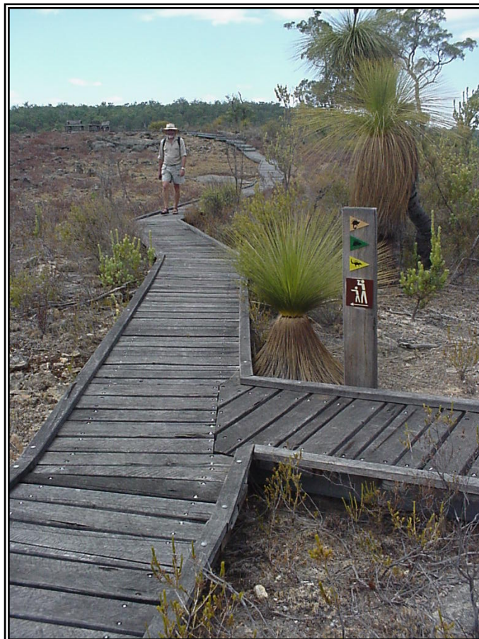
Figure 2: Class 1 Trail - Boardwalk
