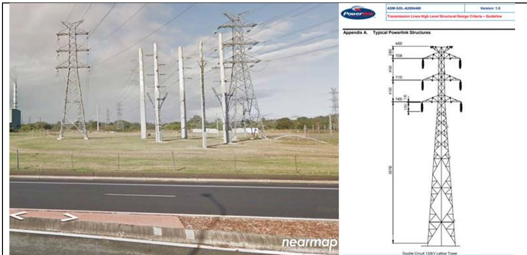
Figure 14: Existing Powerlink Structures in the Brendale area
