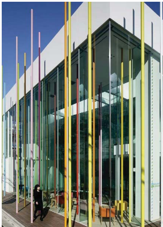
Figure 7. Rainbow mille-feuille Tokyo, by artist Emmanuelle Moureaux. This commercial building is offset 2m from the property line to allow for the installation of 48 coloured sticks on both sides of the glazed facade. Image courtesy of Daisuke SHIMA
