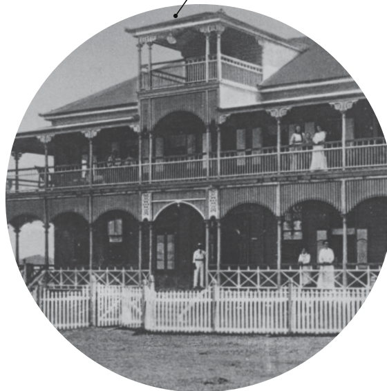
Architectural Elements and Filigree Characterised by delicate filigree Deep eaves and verandah for sun protection Observatory or "widow's walk" for unimpeded views of the sea
