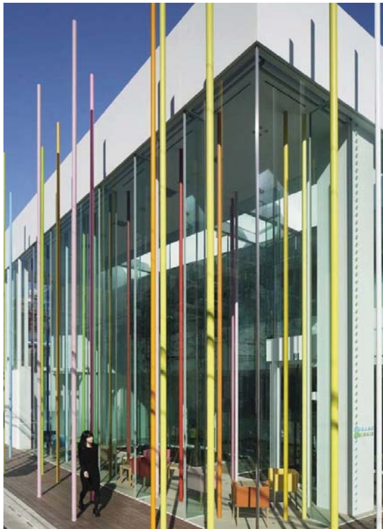
Figure 7. Rainbow mille-feuille Tokyo, by artist Emmanuelle Moureaux. This commercial building is offset 2m from the property line to allow for the installation of 48 coloured sticks on both sides of the glazed facade. Image courtesy of Daisuke SHIMA
