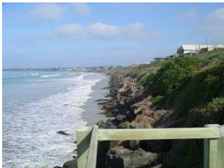
Figure 4-3 Seawalls on eroding shorelines cause loss of usable beach
