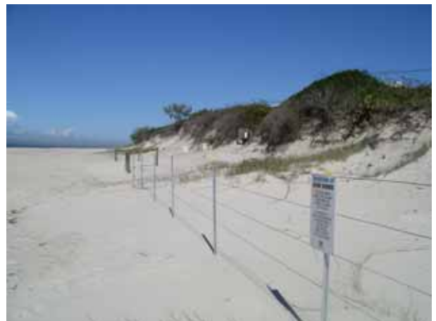
b) Dune fencing to prevent pedestrian access and facilitate Spinifex growth for trapping wind blown sand in the foredune
