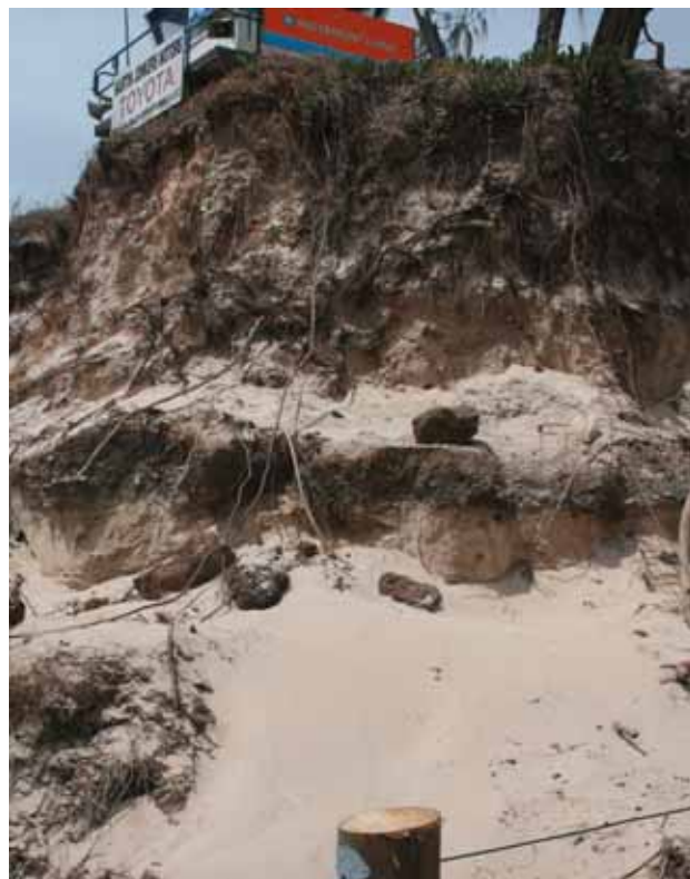
Figure 3-31 Old bitumen surface exposed below wind blown sand and mature vegetation in the eroding dune scarp adjacent to the surf club area
