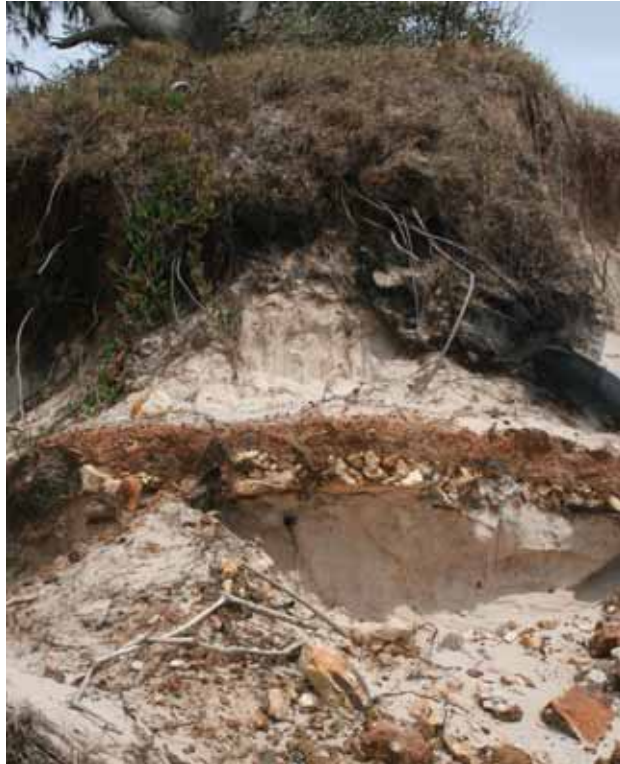
Figure 3-30 Old gravel road base horizon exposed below wind blown sand and mature vegetation in the eroding dune scarp adjacent to the surf club area
