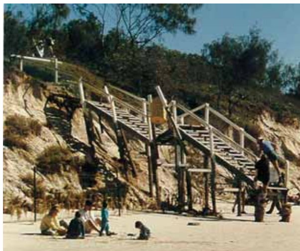
Erosion at stairs near COPE station in 1988
