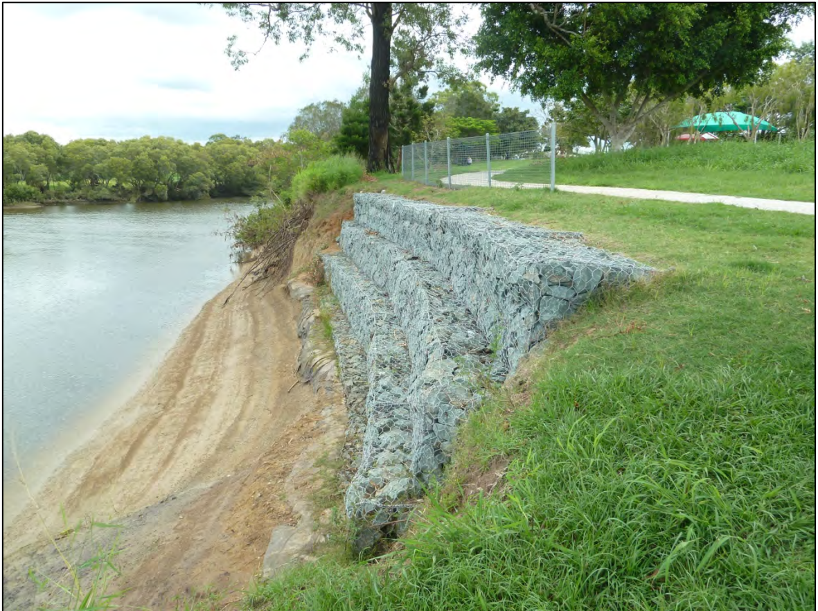
Figure 4-3 Erosion Protection on Normanby Way
