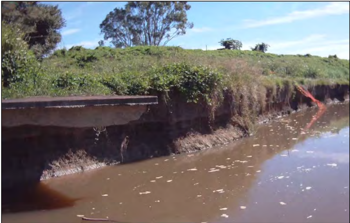
Figure 4-2 Pitonga Way Erosion
