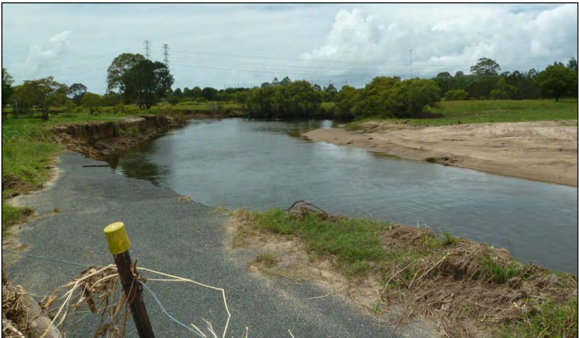
Figure 3-2 Damage to Sealed Bikeway at Pine Rivers Park
