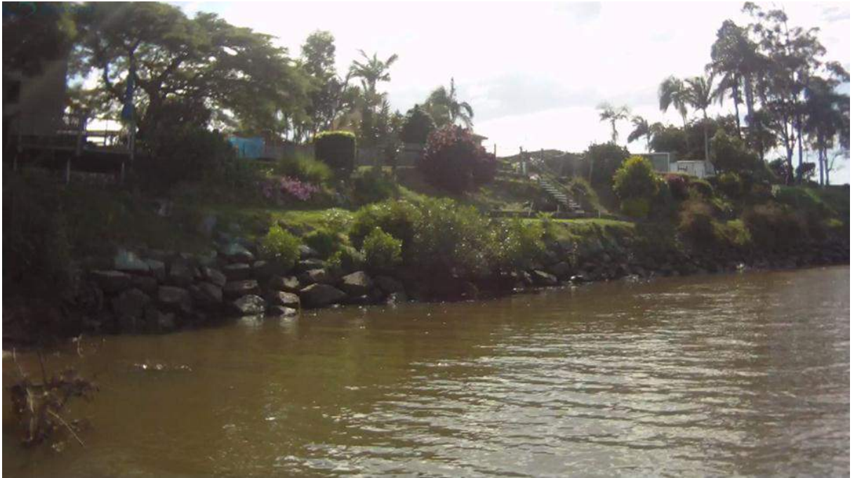
Figure 5-9 Moderate Erosion Risk Example (Learmonth Street)
