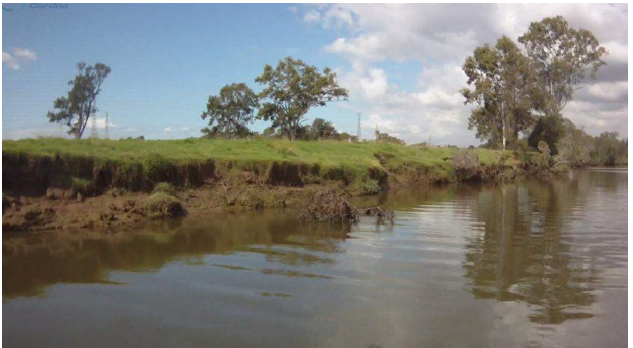
Figure 5-8 High Erosion Risk Example
