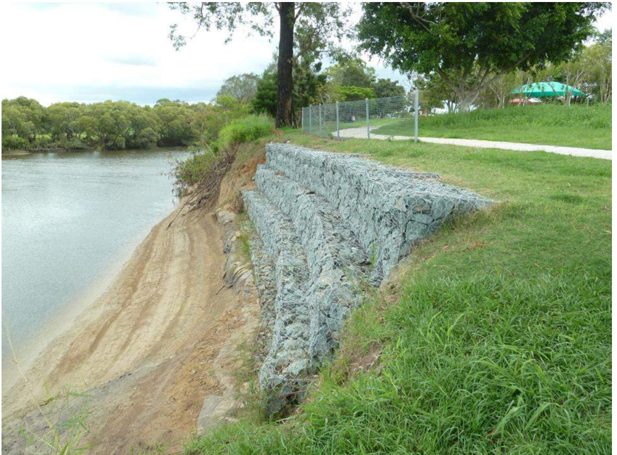
Figure 5-10 Moderate Erosion Risk Example (Pitonga Way)
