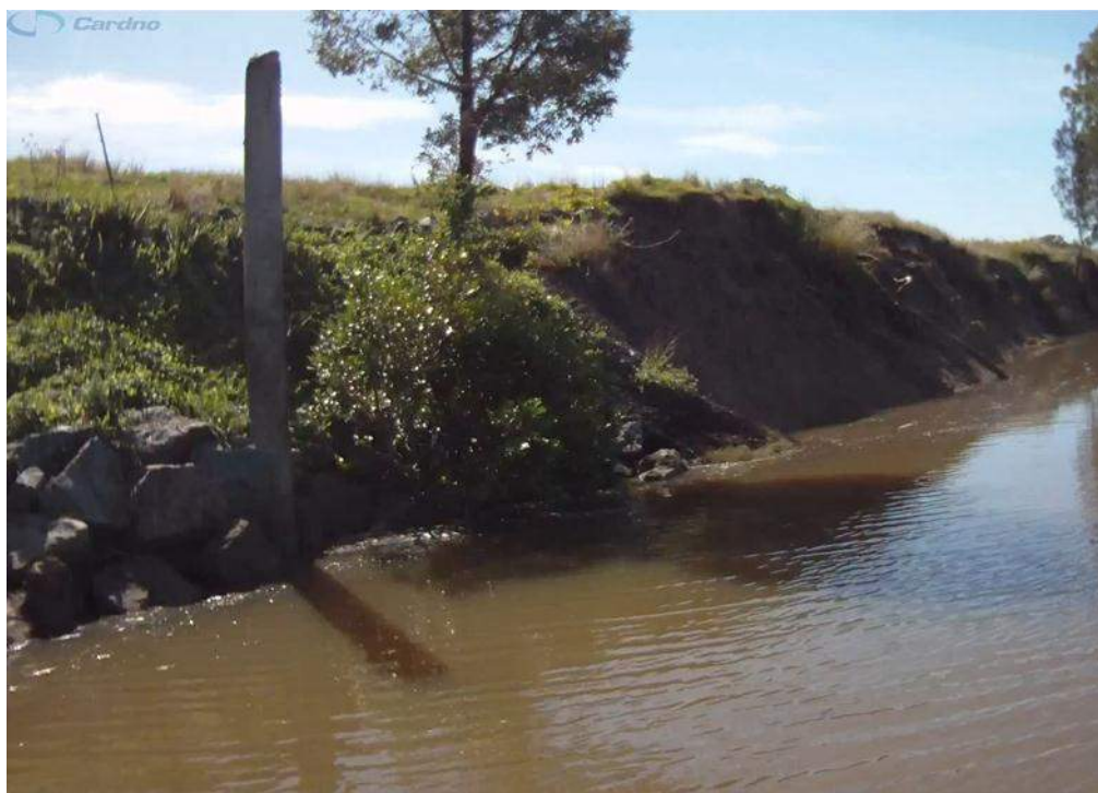
Figure 5-13 Learmonth Street Erosion Protection
