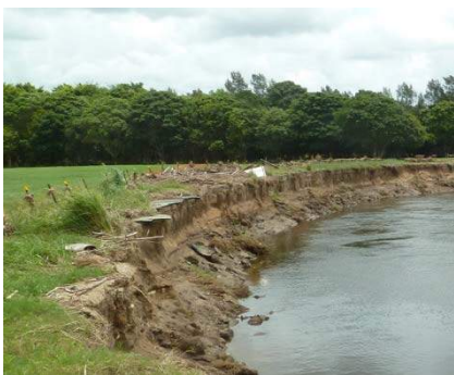
Eroded River Bank at Pine Rivers Park
