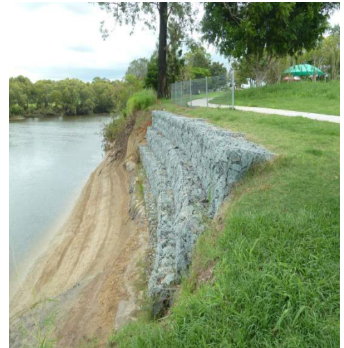
Rock Filled Gabion Retaining Wall on Normanby Way
