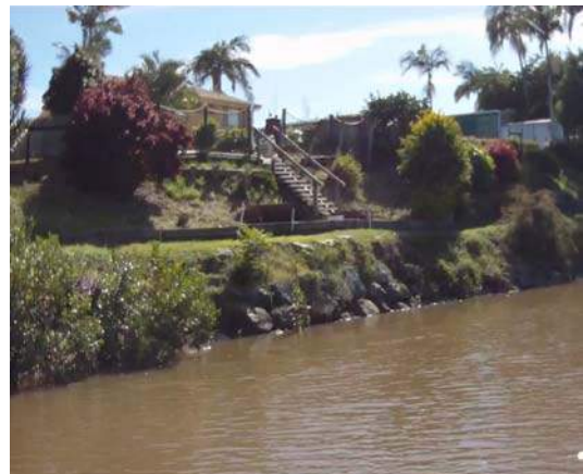
Private Erosion Protection at Learmonth Street
