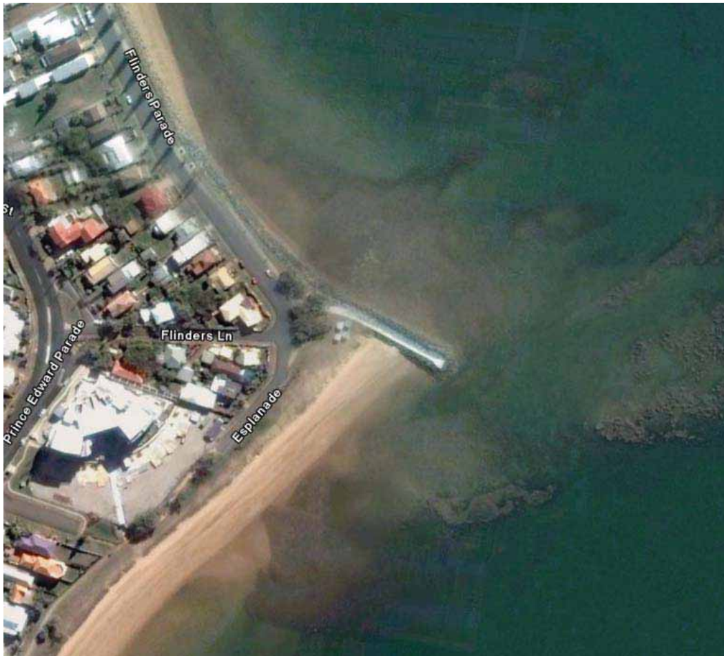
Figure 4-1 Beach at Osbourne Point groyne showing impact of a groyne
