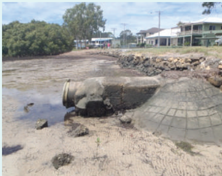
Stone and concrete seawall identified for upgrade (Section 9)
