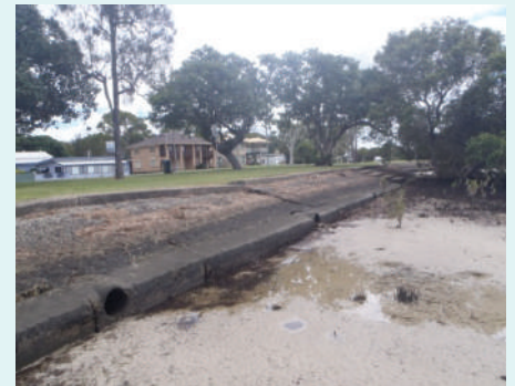
Sloping concrete seawall slumping (Section 10)
