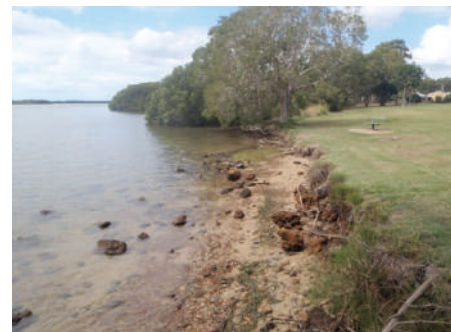
Loose rock and erosion scarp (Section 4)
