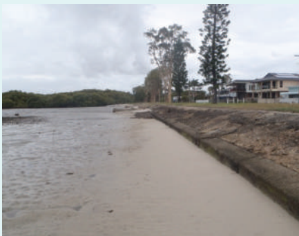
Sloping concrete seawall and narrow beach (Section 1)
