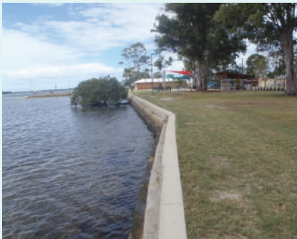
Repaired stepped concrete seawall (Section 5)
