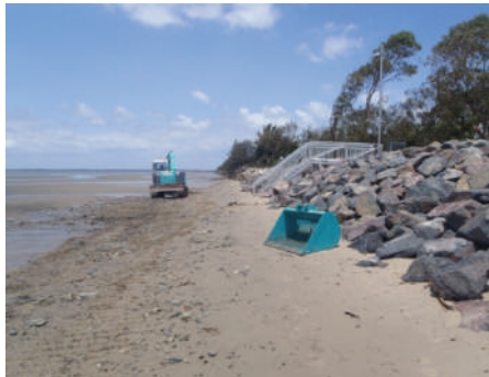
Rock seawall construction at Beachmere Activity Centre
