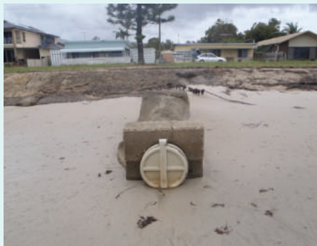
Stormwater outlet with minor sand accumulation on northern side
