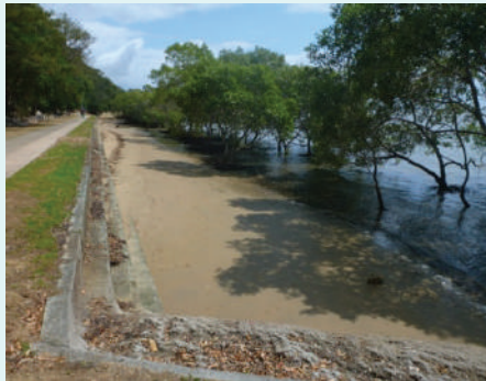
Stepped seawall with mangrove buffer
