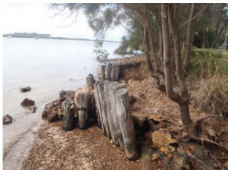
Loosely placed rock and timber (Section 3)
