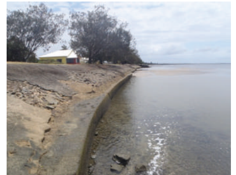
Concrete seawall in poor condition (Section 10)
