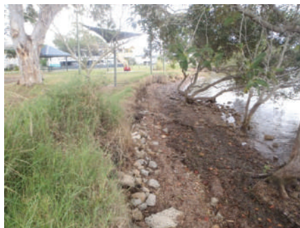
Grassy shoreline and playground equipment (Section 2)
